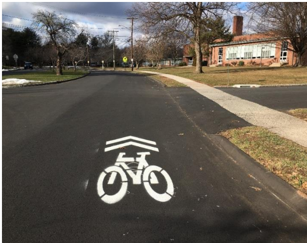
Westminster Drive Sharrow Pavement Marking Looking South towards Duffy Elementary School
