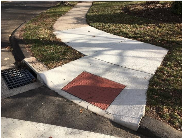
Westminster Drive Sidewalk Ramp Installation
