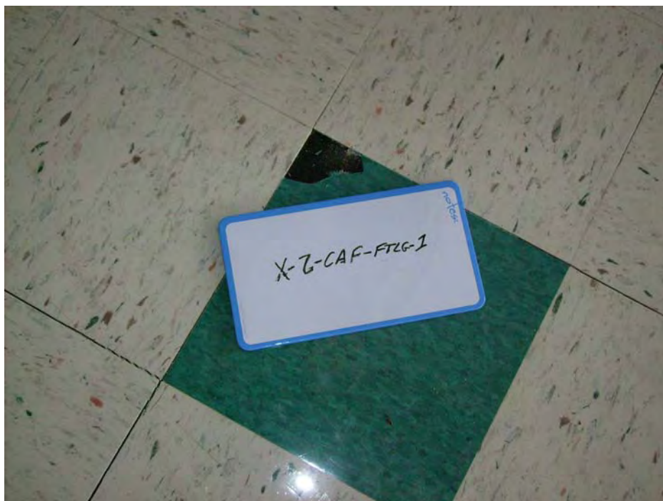
12x12 light green floor tile and associated mastic represented by sample number X-2-CAF-FTLG-1 located in the cafeteria of the Annex Building.
