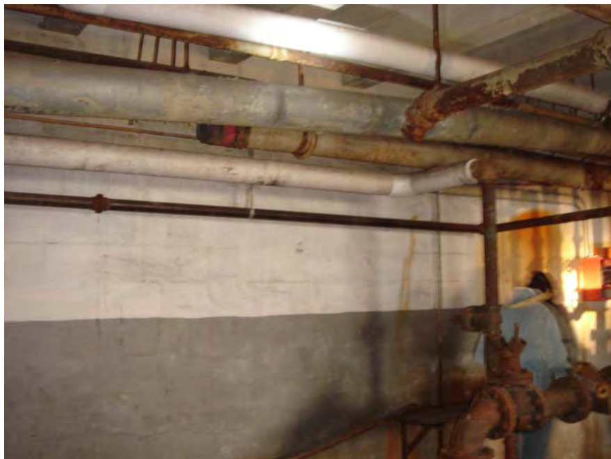
Photo 11: Suspected mold growth on pipes and walls in the lower boiler room in the basement of Building B. Sample MD-B-G-BR-1 was taken here.
