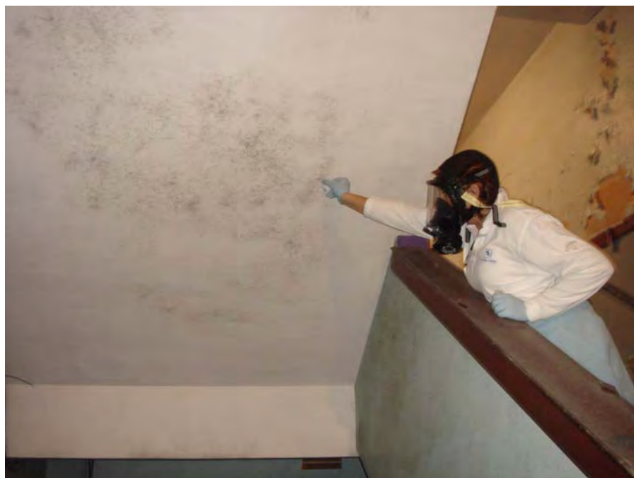
Photo 20: Suspected mold growth on the walls of a stairwell of Building D on the first floor where sample No. MD-D-1-SW-1 was taken.
