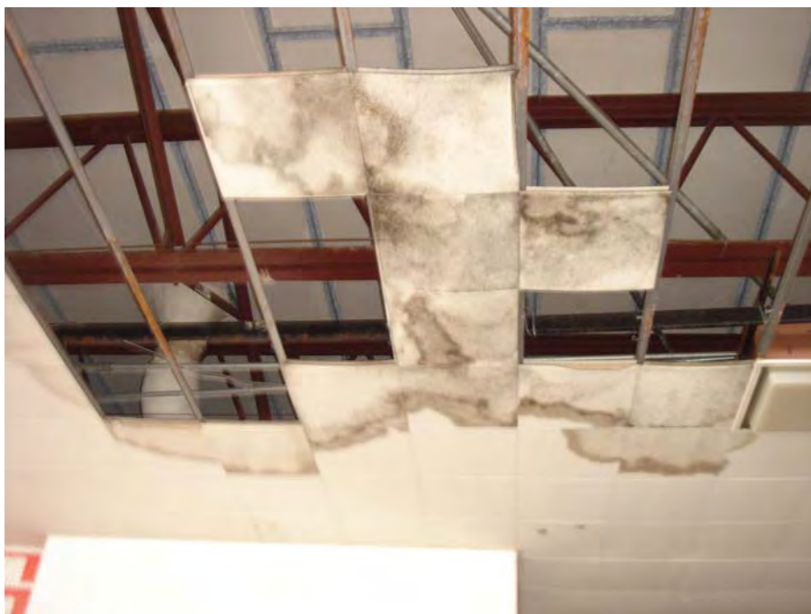
Photo 4: Water damaged ceiling tiles and suspected mold located in a Cafeteria on the third floor of Building A.
