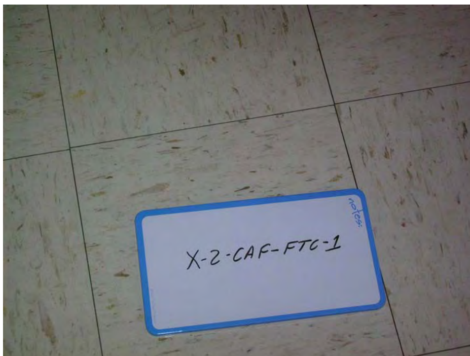
12x12 cream floor tile and associated mastic represented by sample number X-2-CAF-FTC-1 located in the cafeteria of the Annex Building.
