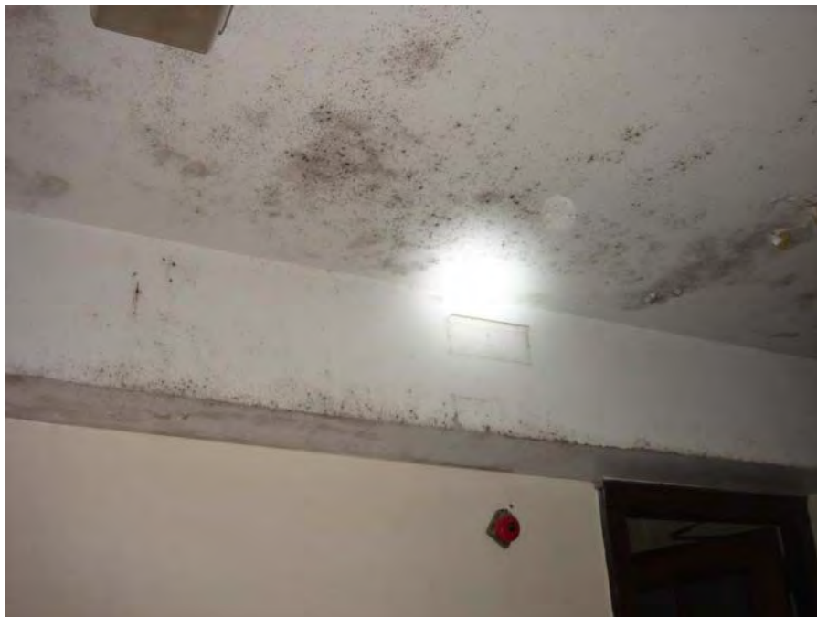
Photo 9: Suspected mold growth on the ceiling and walls of the pool locker room in Building B on the basement floor. Sample MD-B-LR-1 was taken here.
