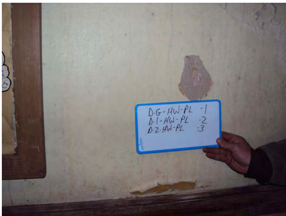
Plaster represented by sample numbers D-G-HW-PL-1, D-1-HW-PL-2 and D-2-HW-PL-3 located on the ground, 1 st and 2 nd floor of Building D.
