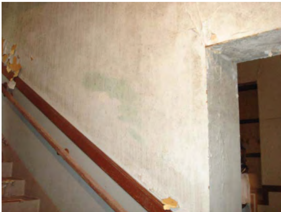
Photo 15: Suspected mold growth on the walls of a stairwell of Building C on the first floor where sample No. MD-C-1-SW-1 was taken.
