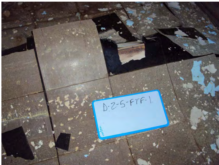
Floor tile felt represented by sample number D-2-5-FTF-1 located on the 2 nd floor of Building D.
