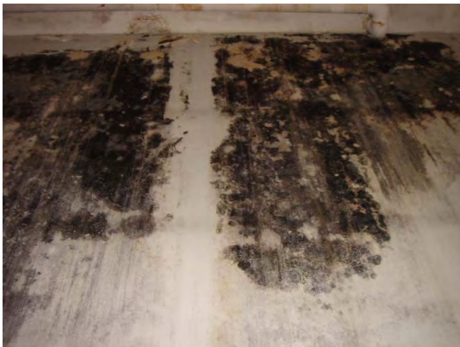
Photo 6: Suspected heavy black mold growth on the south wall of the south classroom on the second floor in Building A.
