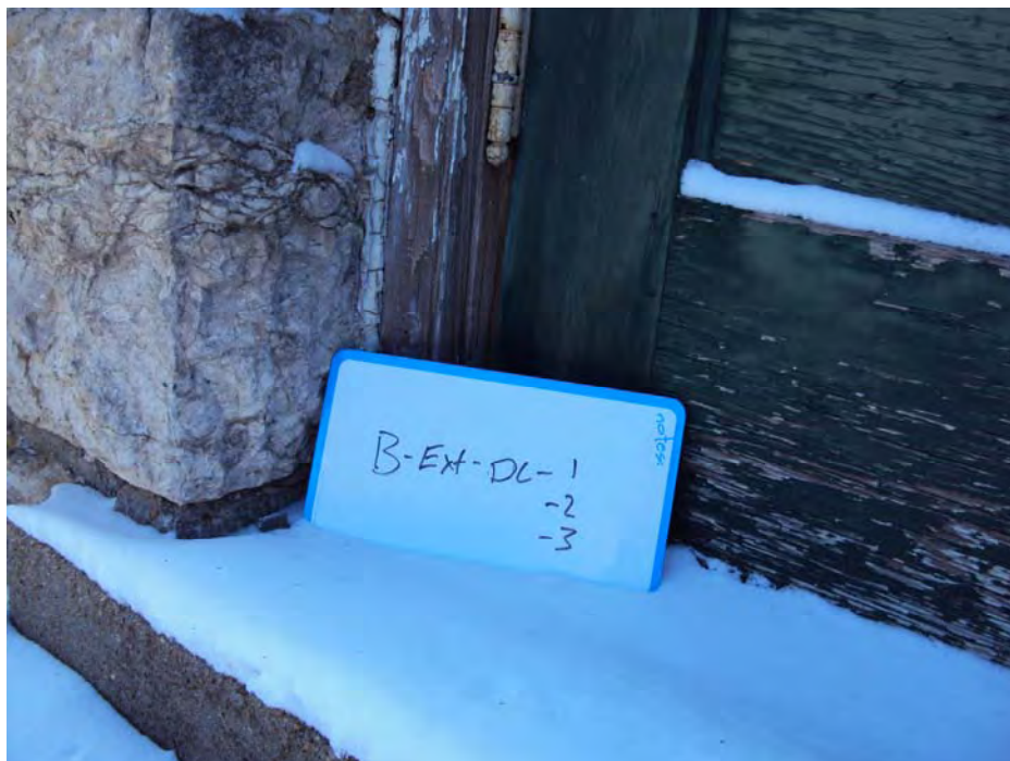
Exterior door caulking represented by sample numbers B-EXT-DC-1, 2 and 3 located on the exterior doors of Building B.
