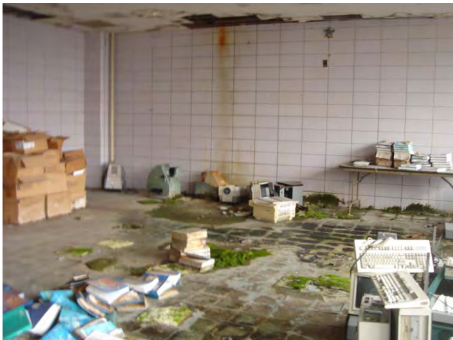
Photo 3: Suspected mold growth in Cafeteria of Building A on the third floor.
