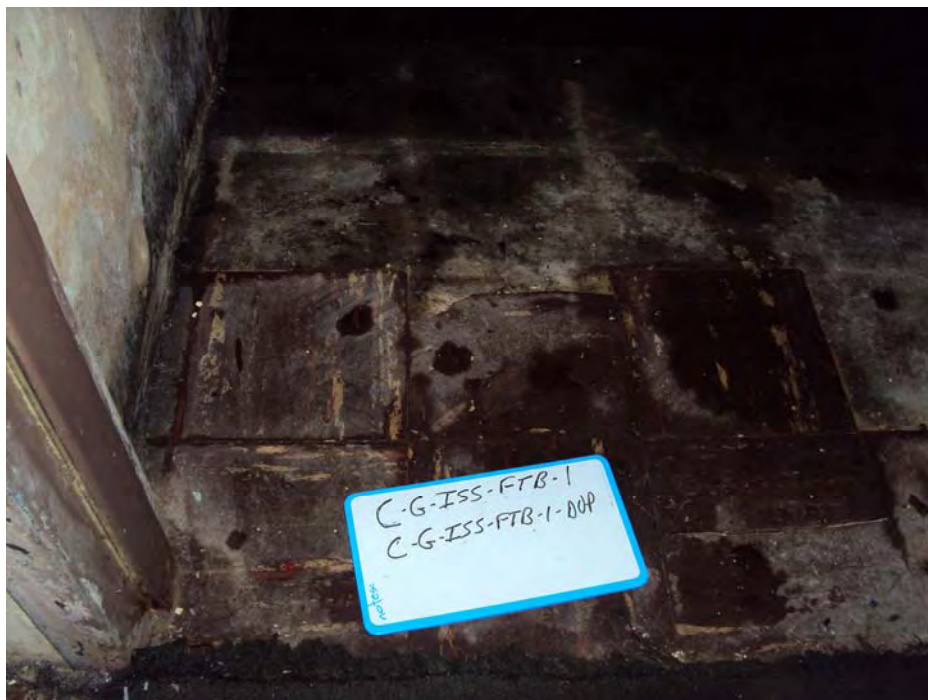
12x12 brown floor tile and associated mastic represented by sample numbers C-G-ISS-FTB-1 and C-G-ISS-FRB-1-DUP located in the ISS room of Building C.
