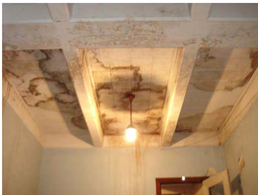
Photo 22: Suspected mold growth on the walls and ceilings on the second floor of Building D where sample No. MD-D-2-SW-1 was taken.
