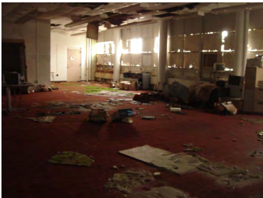
Photo 7: Suspected mold growth and water damage in the west classroom on the second floor of Building A.
