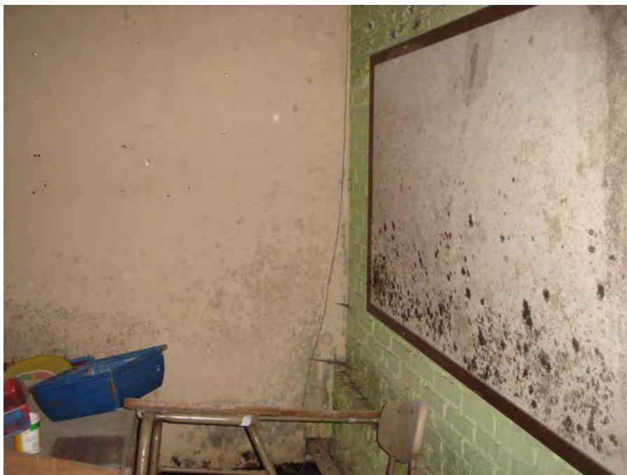
Photo 16: Suspected mold growth on the walls of Room 19 in Building C on the ground floor where sample No. MD-C-G-19-1 was taken.
