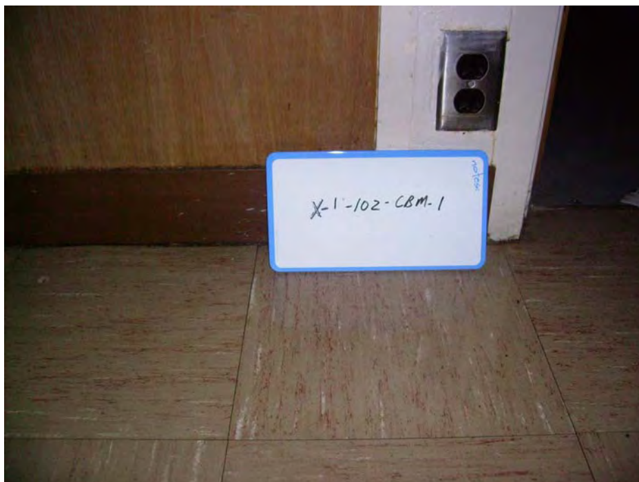
Cove base mastic represented by sample number X-1-102-CBM-1 located in room 102 of the Annex Building.
