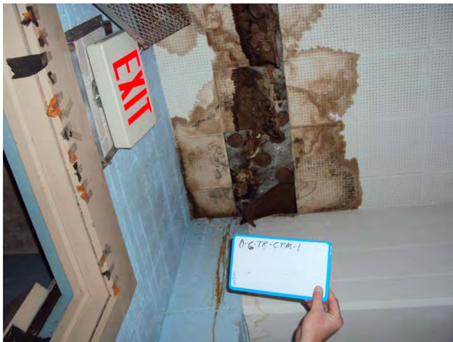
Ceiling tile mastic represented by sample number D-G-TR-CTM-1 located in the transition room of Building D.
