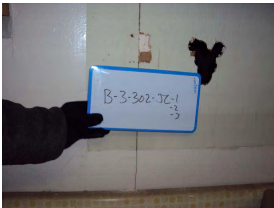
Joint compound represented by sample number B-3-302-JC-1, 2 and 3 located in room 302 of Building B.
