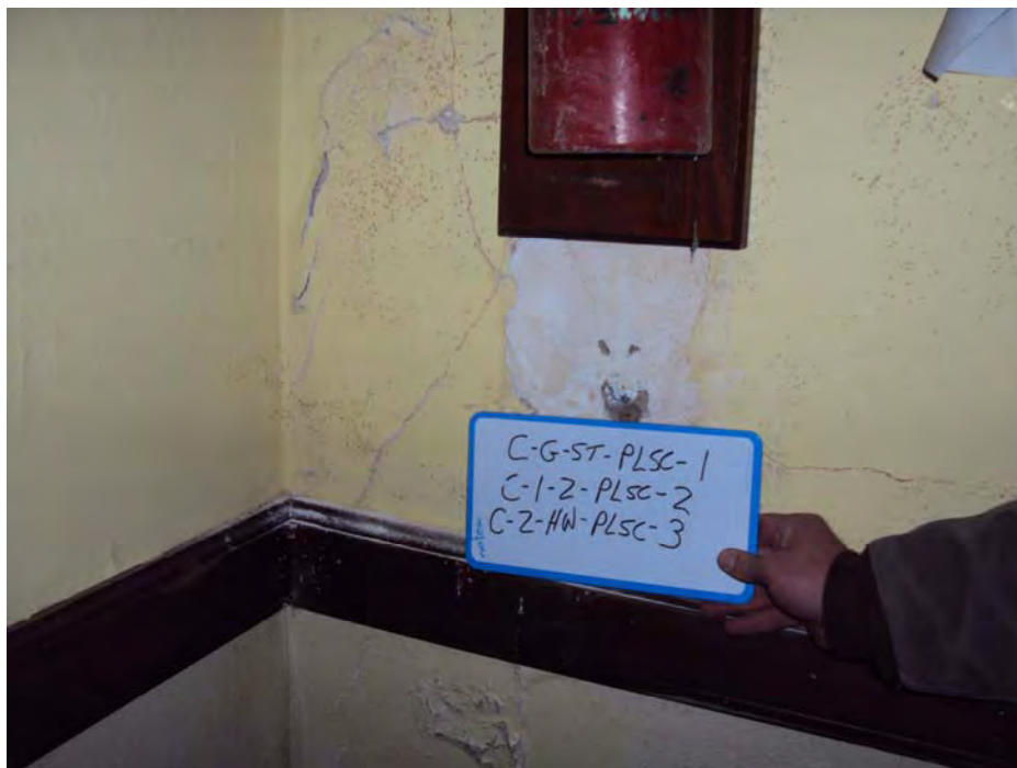
Plaster skim coat represented by sample numbers C-G-ST-PLSC-1, C-1-2-PLSC-2 and C-2-HW-PLSC-3 located on the ground, 1 st and 2 nd floor of Building C.
