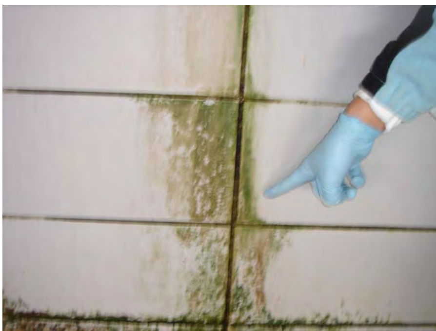
Photo 2: Suspected mold growth in Cafeteria, third floor of Building A, where sample No. MD-A-3-CAF-1 was taken.
