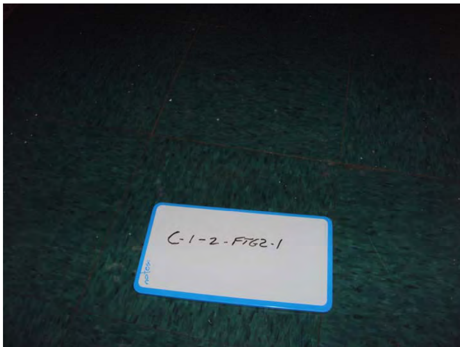
12x12 dark green floor tile and associated mastic represented by sample number C-1-2-FTG2-1 located in room 2 of Building C.
