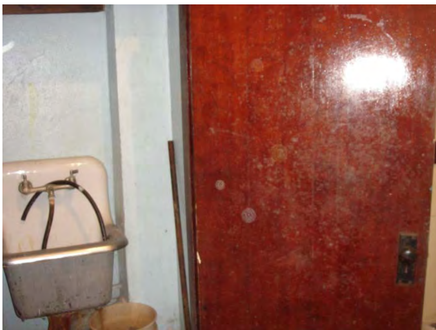
Photo 14: Suspected mold growth on the door of a janitor's closet in the hallway on the second floor in Building C. Sample No. MD-C-2-CL-1 was taken here.
