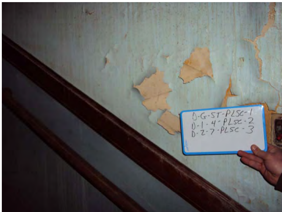
Plaster skim coat represented by sample numbers D-G-ST-PLSC-1, D-1-4-PLSC-2 and D-2-7-PLSC-3 located on the ground, 1 st and 2 nd floor of Building D.
