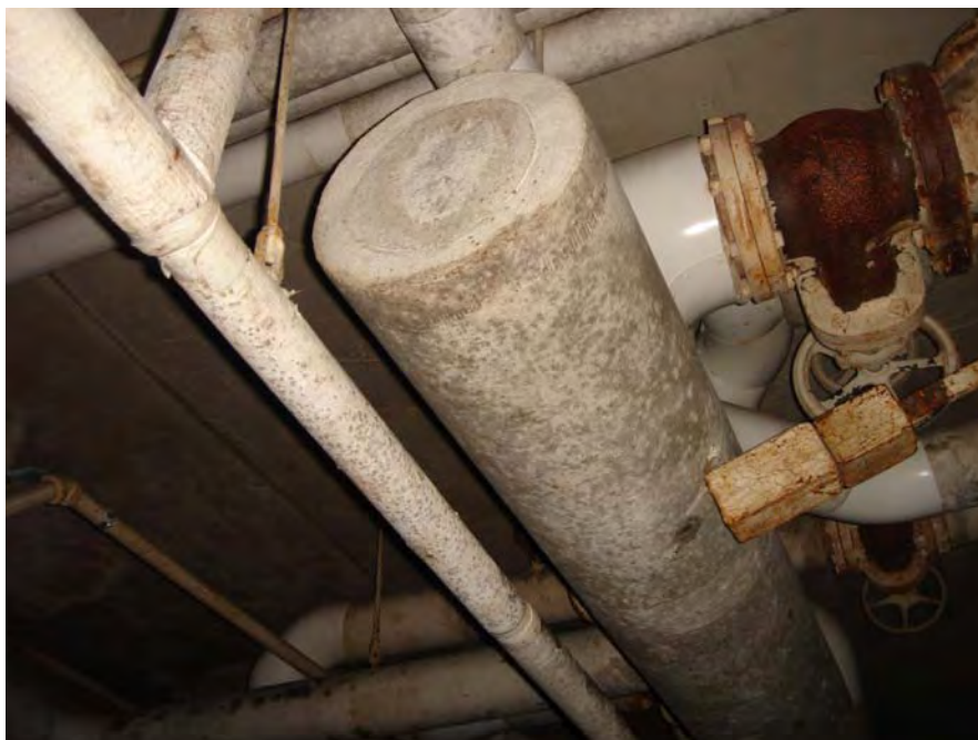
Photo 17: Suspected mold growth on the ceiling and pipes on the ground level of Building C, where sample No. MD-C-G-Mech-1 was taken.
