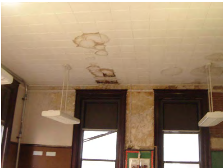
Photo 13: Water damaged ceiling tiles in Room 11 on the second floor of Building C.
