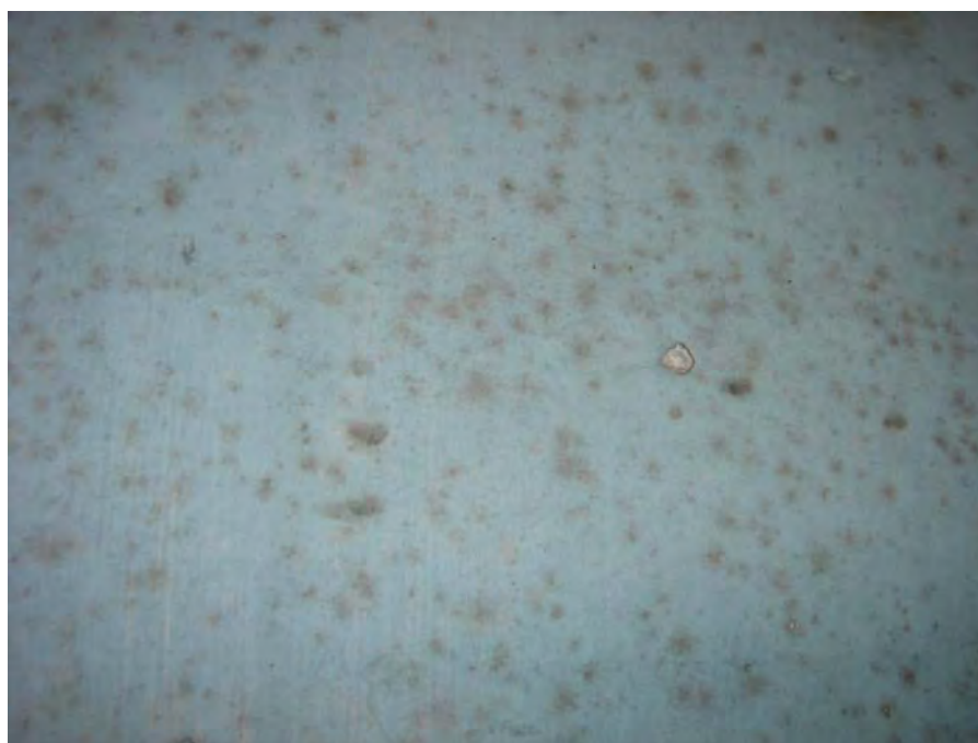
Photo 18: Suspected mold growth on the walls of the Transition Center in Building D on the ground floor where samples MD-D-G-TR-1 and MD-D-G-TR-1DUP were taken.
