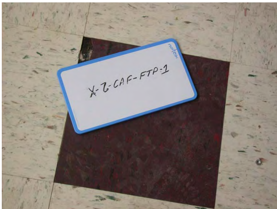
12x12 purple floor tile and associated mastic represented by sample number X-2-CAF-FTR-1 located in the cafeteria of the Annex Building.
