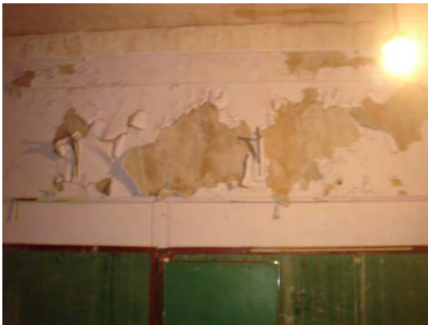
Photo 21: Water damage on the walls and ceiling in Room 8 on the north side of the building in Building D.
