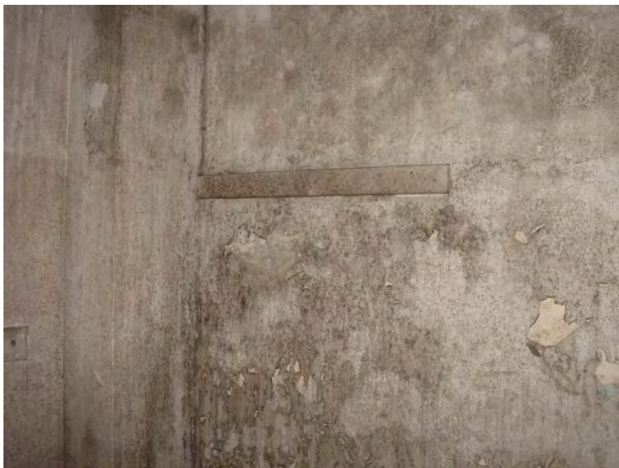
Photo 10: Suspected mold growth on the ceiling and walls of the pool locker room in Building B on the basement floor.
