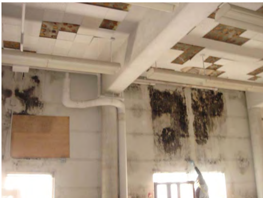
Photo 5: Suspected mold growth on the south wall of the south classroom on the second floor in Building A where samples MD-A-2-SR-1 and MD-A-2-SR-1DUP were taken.
