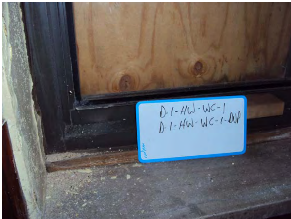
Window caulking represented by sample numbers D-1-HW-WC-1 and D-1-HW-WC-1-DUP located on the 1 st floor of Building D.
