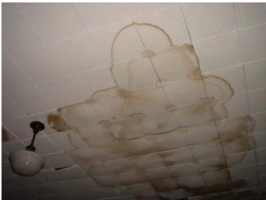
Photo 12: Water damaged ceiling in the auditorium on the ground floor in Building B.
