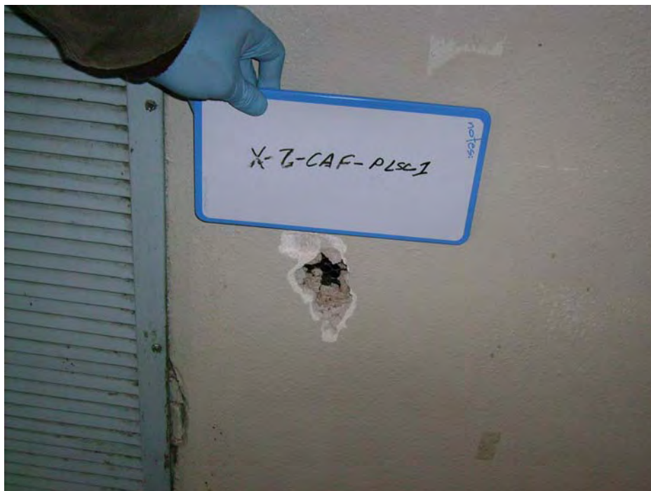
Plaster skim coat represented by sample number X-2-CAF-PLSC-1 located in the cafeteria of the Annex Building.
