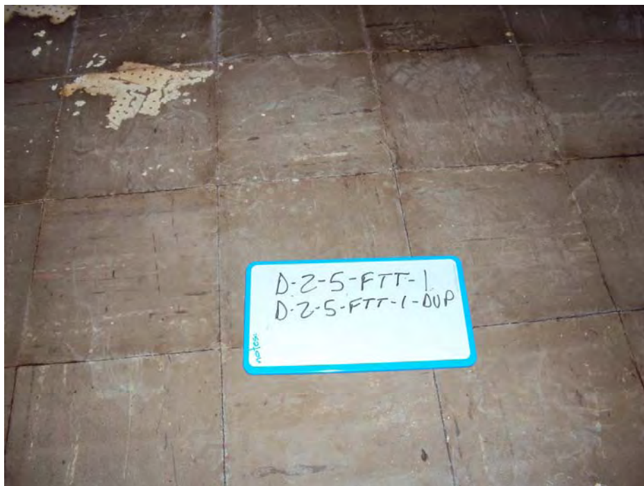
12x12 tan floor tile and associated mastic represented by sample numbers D-2-5-FTT-1 and D-2-5-FTT-1-DUP located on the 2 nd floor of Building D.
