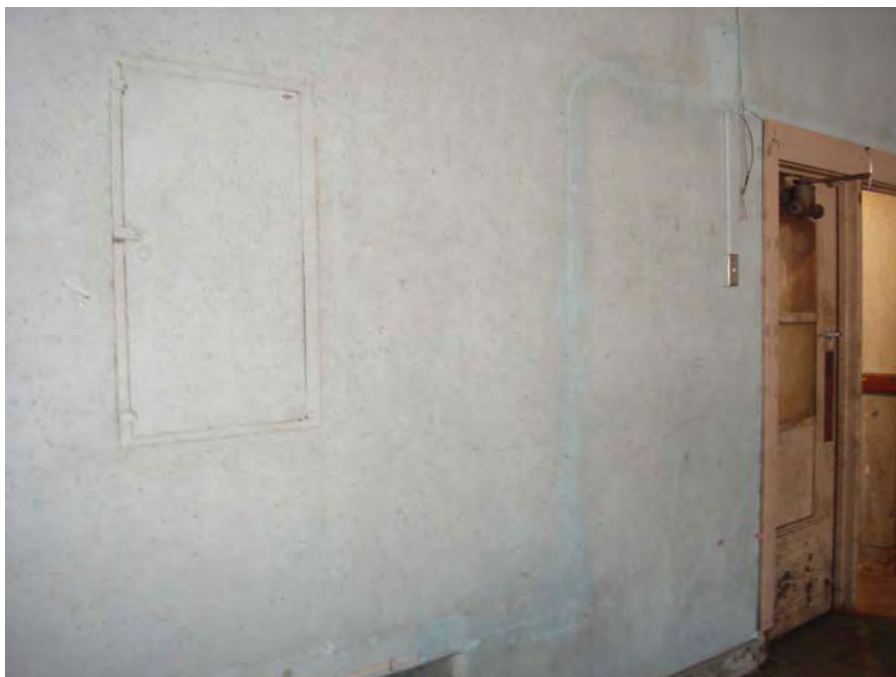
Photo 19: Suspected mold growth on the walls of the Transition Center in Building D on the ground floor where samples MD-D-G-TR-1 and MD-D-G-TR-1DUP were taken.
