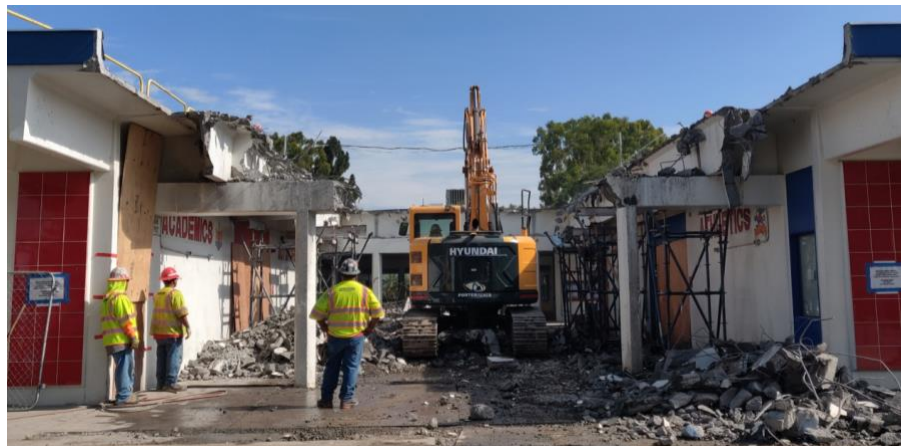
Demolition of the breezeway entrance to Los Alamitos High.
