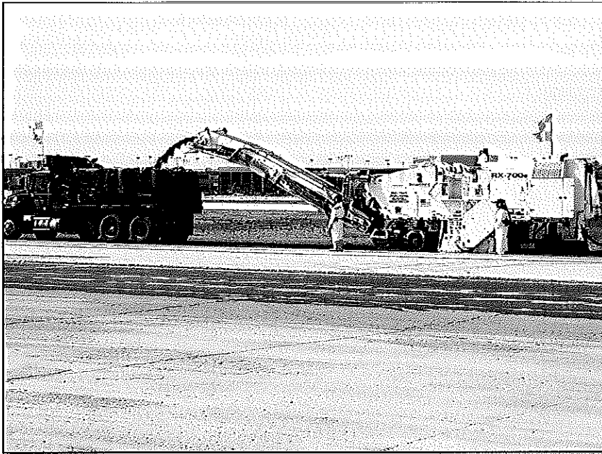
Philadelphia International Airport (PHL); removal of asbestos-containing asphalt from runway.
