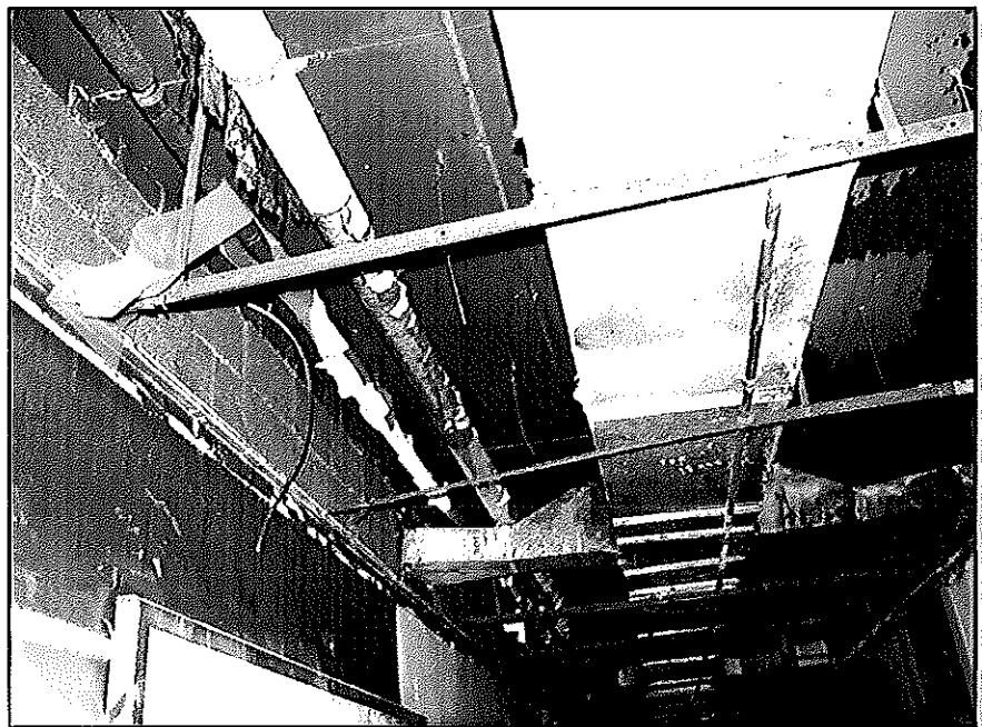
Asbestos materials impacted by fire, too.
