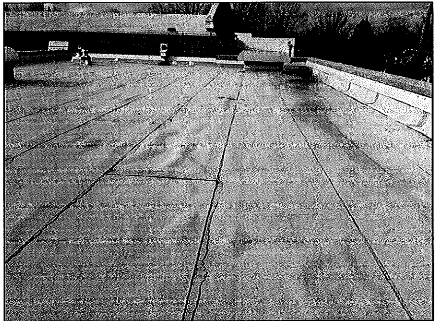
Roof damage allowed moisture into building into gym.
