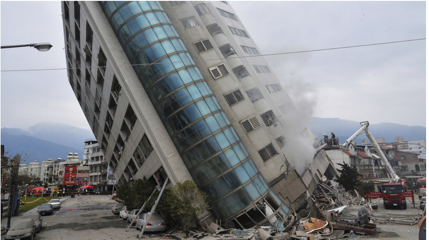
Image 1. A building leans on a collapsed first floor following an earthquake in Hualien, Taiwan, February 7, 2018. Photo: Central News Agency via AP
