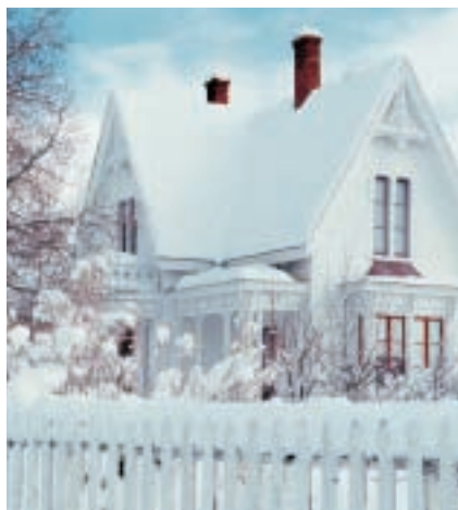
Pitched-roof house, Connecticut
