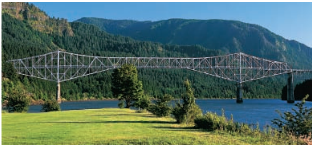
Steel truss bridge over the Columbia River Gorge in Oregon
