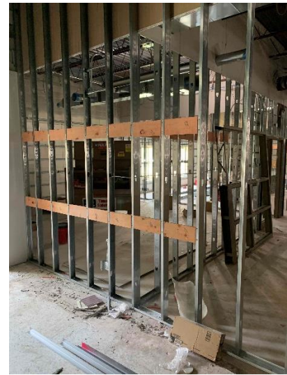
CCES – Electrical rough ins complete in area D
