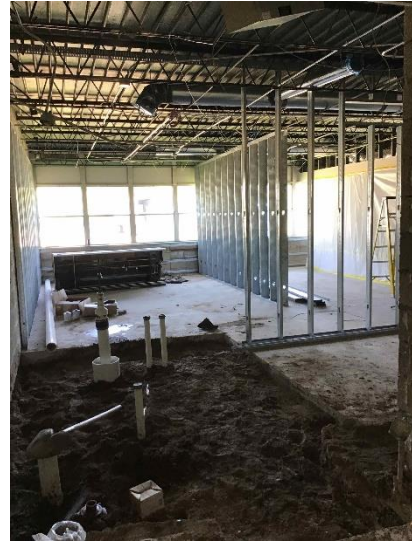
ECFC – underground plumbing in area B classrooms
