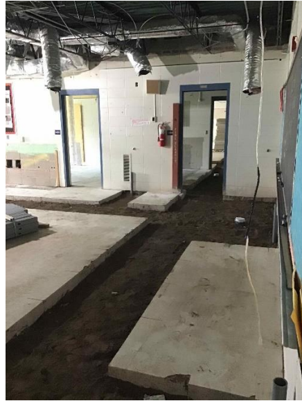
SFMS – Underground plumbing complete in area E classrooms
