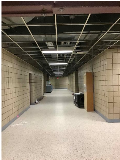
CCES – Ready for new lighting and tiles in area B hallways
