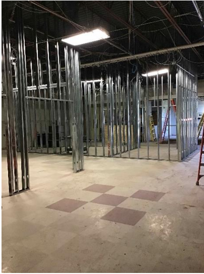
ECFC – new walls being framed in area A
