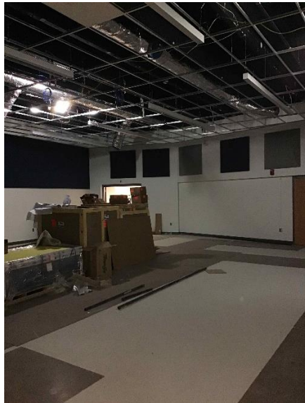
SFHS – Acoustical wall panels installed in area F
