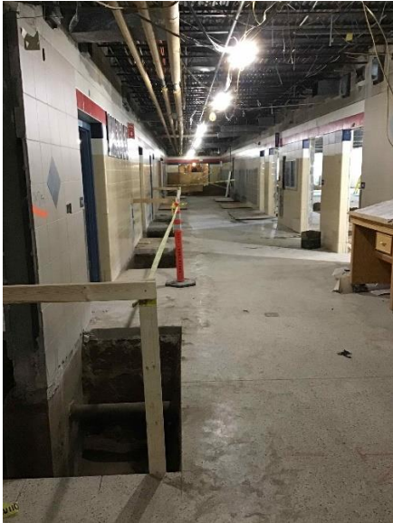
SFMS – Ready for shoring of walls in area D hallways
