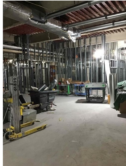
SFHS – Walls being framed in upper area J
