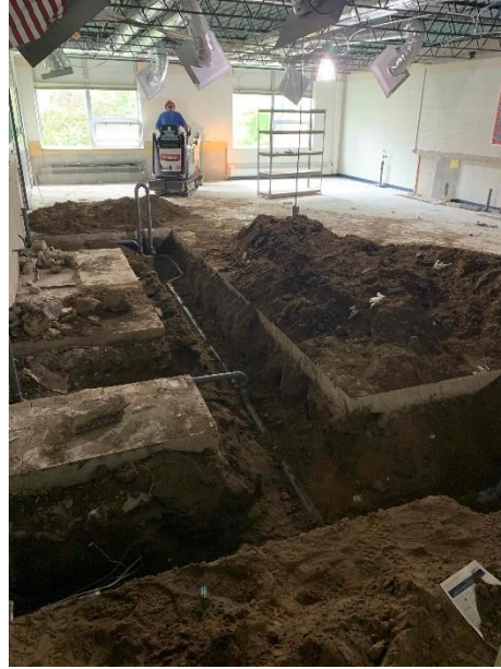
SFMS - sawcut and demo of underground plumbing in area E
