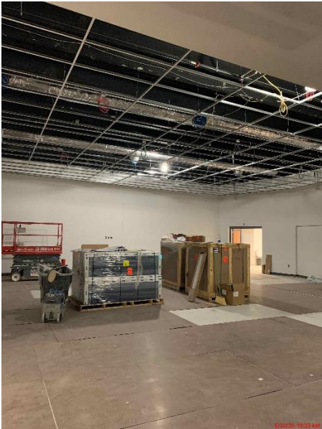
SFHS – Install ceiling grid in area F
