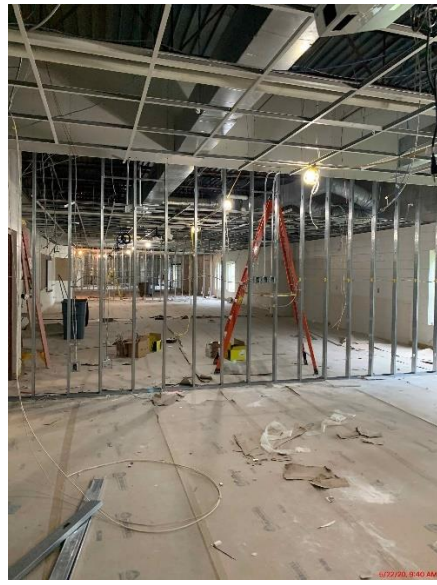
CCES – Finished wall framing in area A classrooms
