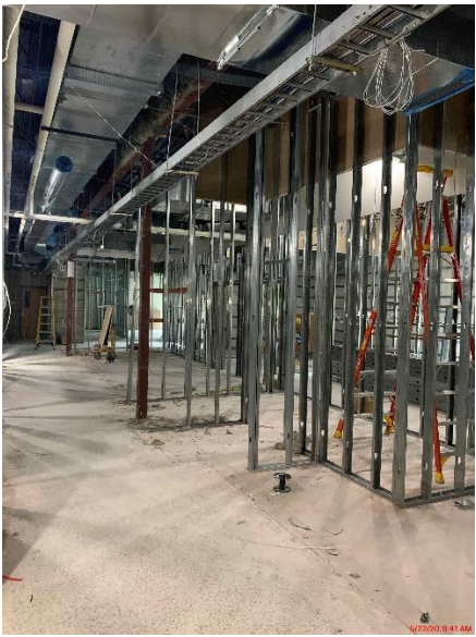
CCES – Finished wall framing in area D - SPED suite
