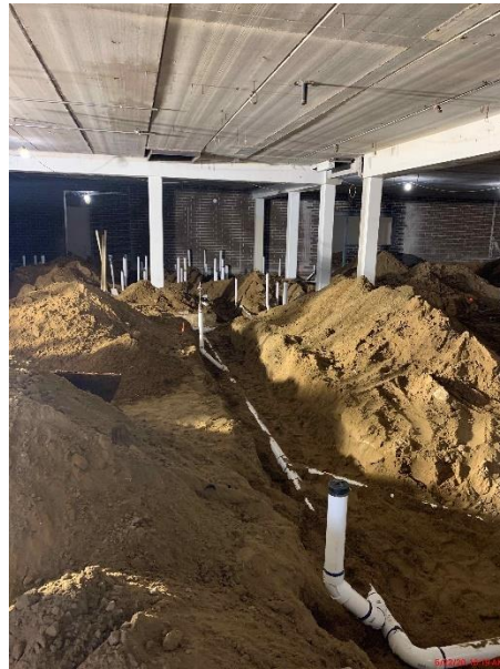
SFHS – underground plumbing in area A locker rooms
