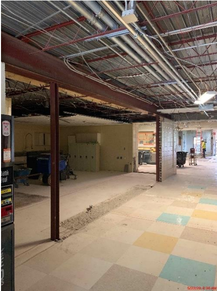
ECFC – Removal of wall and coiling door in area A
