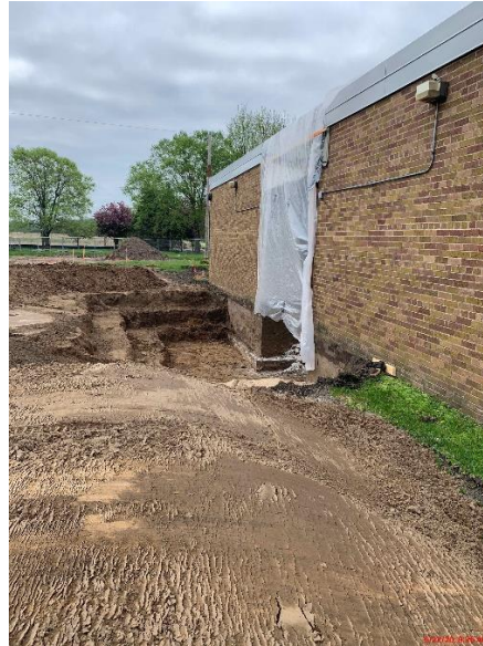
ECFC – Preparation for new stoop on North side of building
