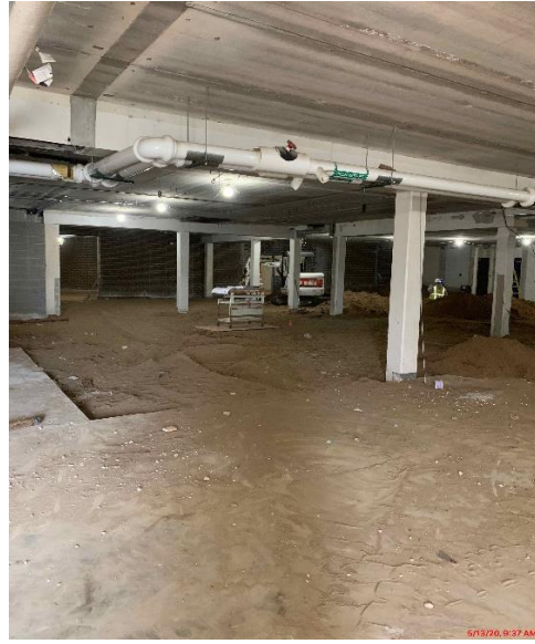
SFHS – Locker room in Area A ready for underground plumbing
