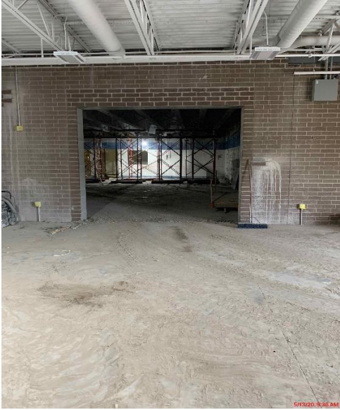
SFHS – Fitness center demo and shoring
