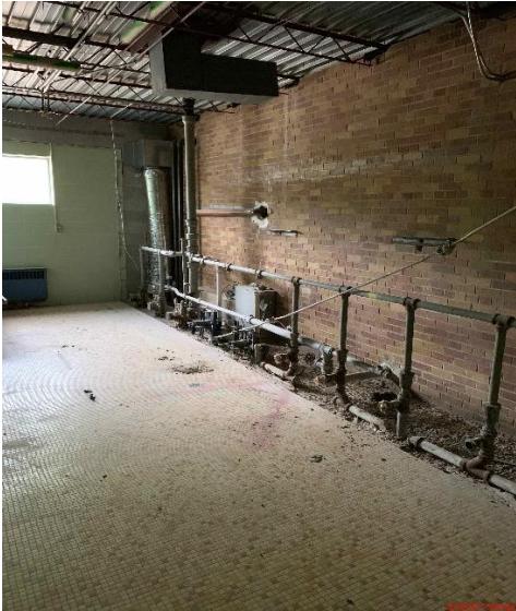
ECFC – demo of bathrooms and plumbing fixtures
