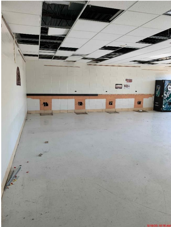
SFMS – Demo of plumbing, casework, and mechanical in Area D
