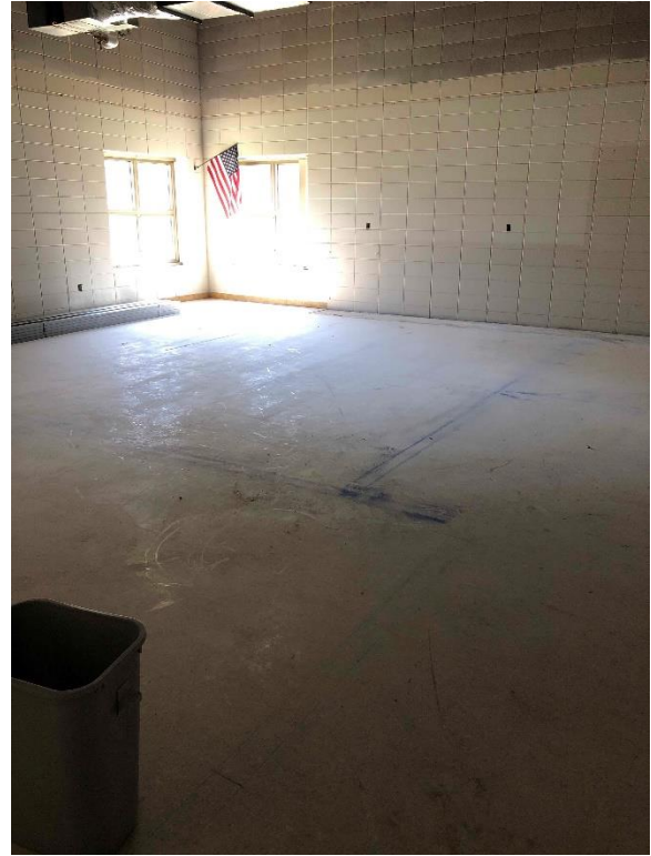
CCES – Prepping for metal wall installation in Area D
