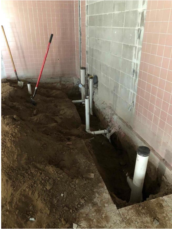
CCES – Saw cutting for plumbing rough-in in Area D
