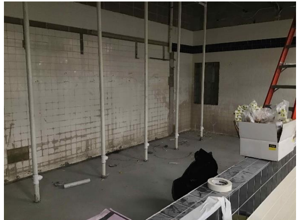
SFMS – Concrete finished in gym locker rooms
