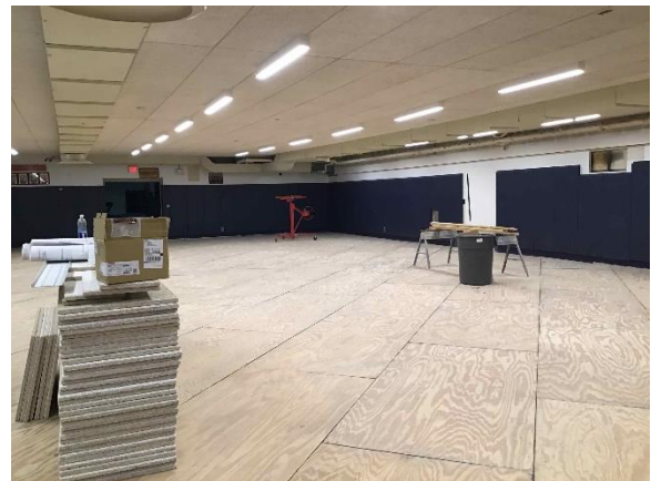
SFHS – Wrestling room ceiling tiles installed
