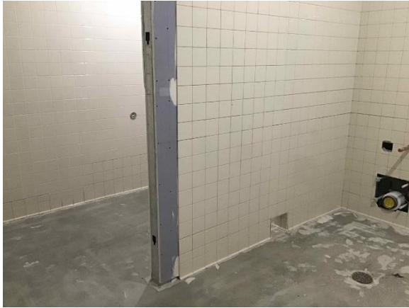
SFMS – ceramic tile being installed in bathroom in upper Area A
