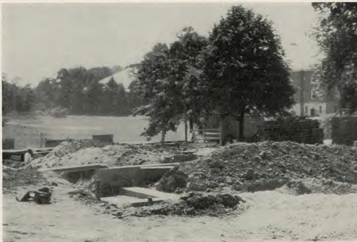
Auditorium Readied For Cornerstone
