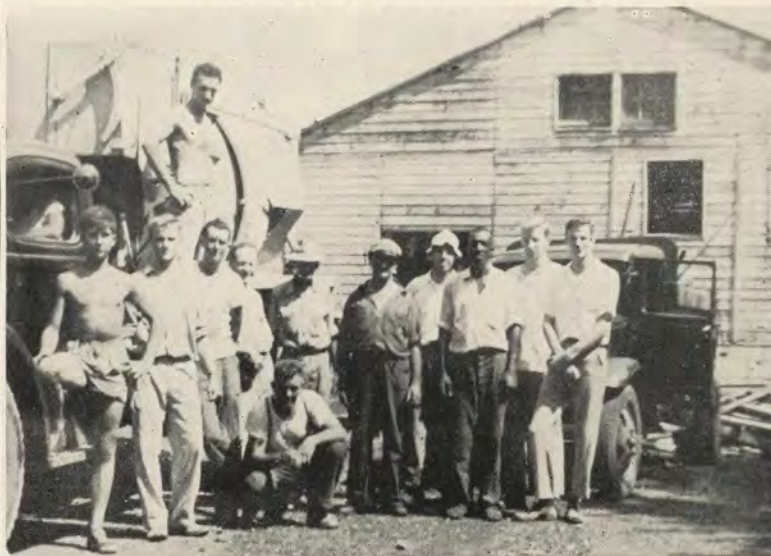
AT GILMAN. During the summer months, a number of Gilman students and faculty re-assembled the prefabricated buildings. Working from the early part of June through most of August, those shown above erected the buildings in back of the main building near the cottage. Since this picture was taken, the new structure has been painted white, windows have been put in, and electricity has been installed.
