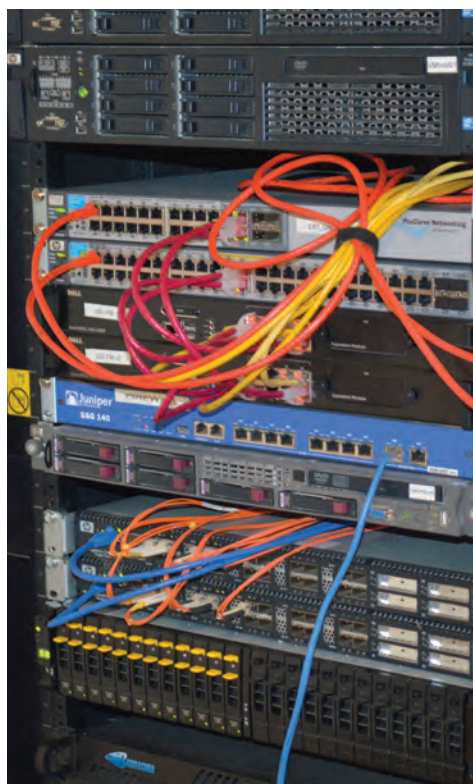
A rack of server equipment in the school's data center. Photo by Luke Wulff
