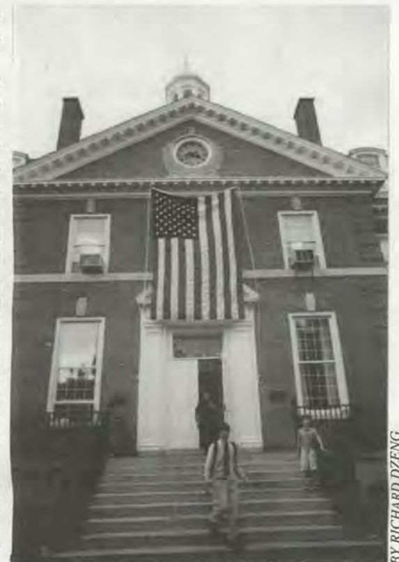
Carey Hall classrooms lack air conditioning.
