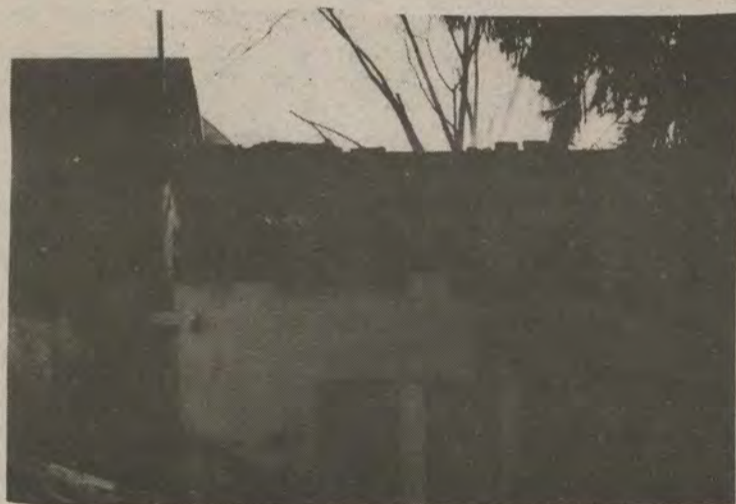
The fire destroyed the entire Lower School.
