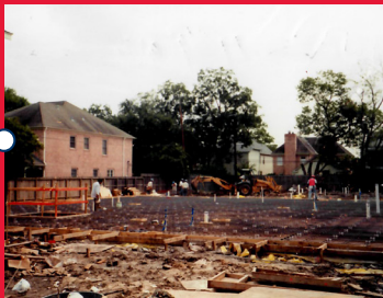
Preparation for building primary school
