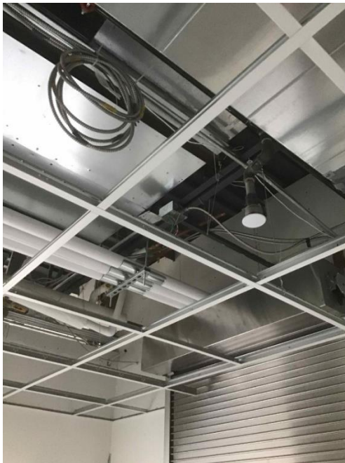
SFHS School Store Grid Install
