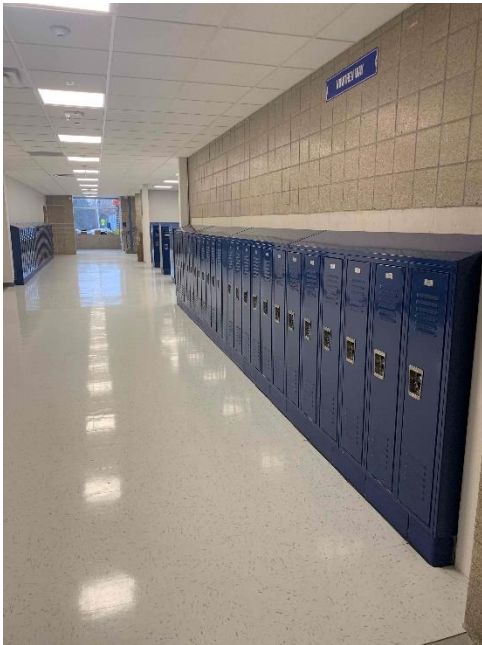
SFMS Lower A Lockers Installed
