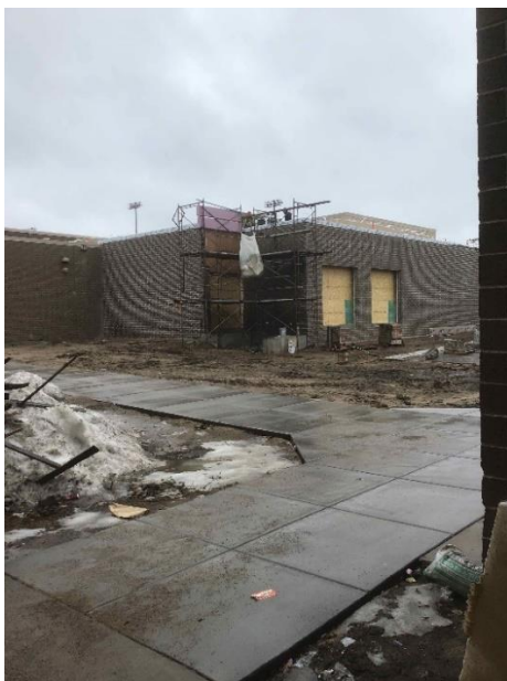
SFHS Fitness Room Exterior Brickwork
