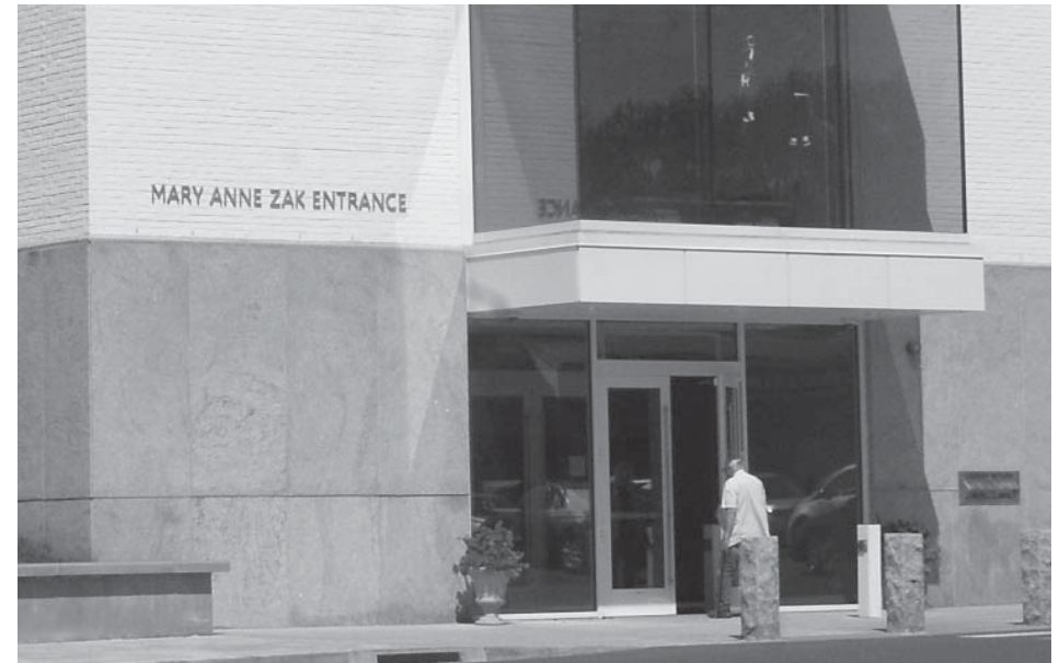
The new entrance provides easy access to the main part of the library via an elevator and stairs.
