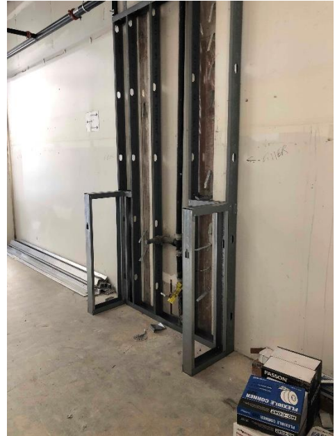
SFMS area A water fountain rough-in
