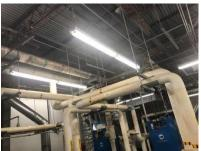
30 High Bay Gym Fixtures (Install new fixtures to bottom of the bar joist)
