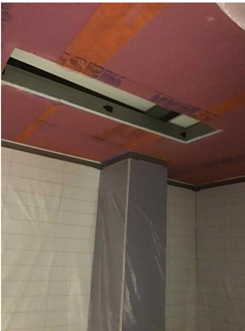
SFHS ceiling install
