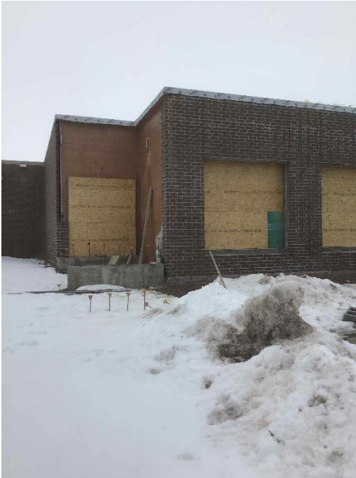
SFHS Weight room window openings
