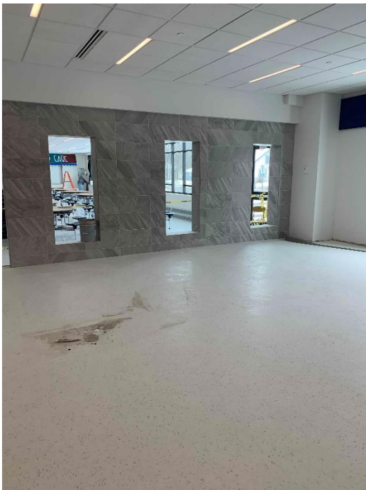
SFMS cafeteria addition paint and tile
