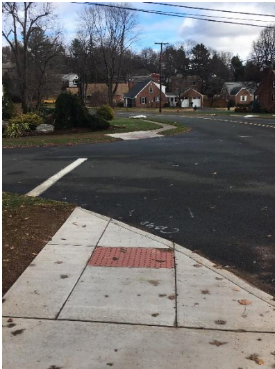
Mountain Road at Tunxis Road Sidewalk Ramp Replacement
