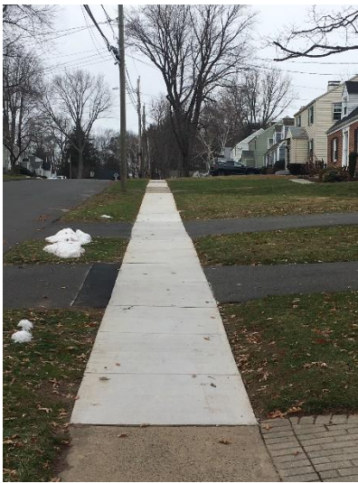
Hilltop Drive Sidewalk Replacement
