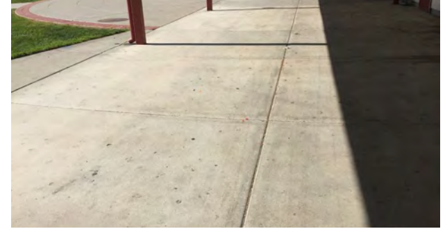
Typical Concrete Paving
