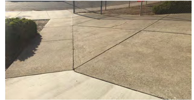
Typical Concrete Paving
