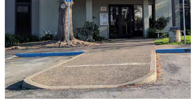
Typical Concrete Paving
