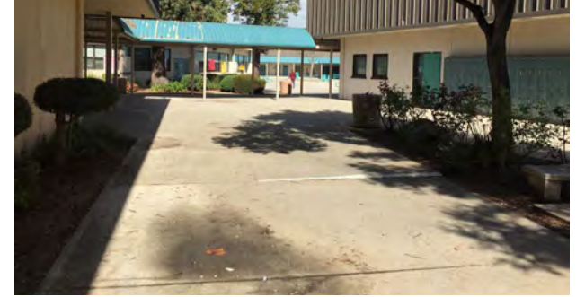
Typical Concrete Paving
