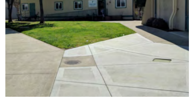
Typical Concrete Paving
