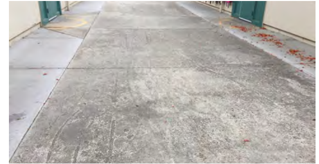
Typical Concrete Paving
