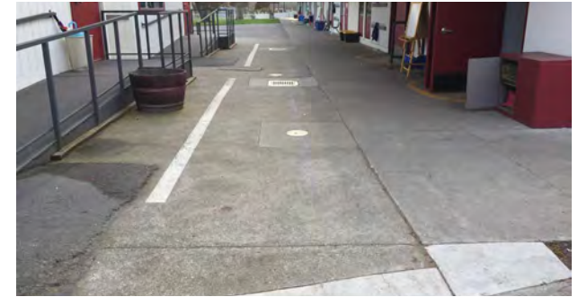
Typical Concrete Paving
