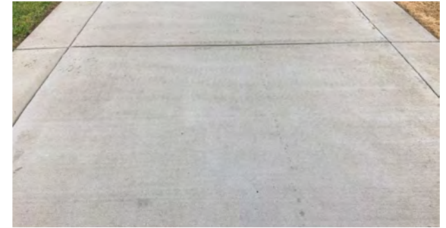
Typical Concrete Paving
