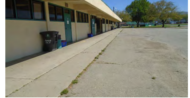
Typical Concrete Paving
