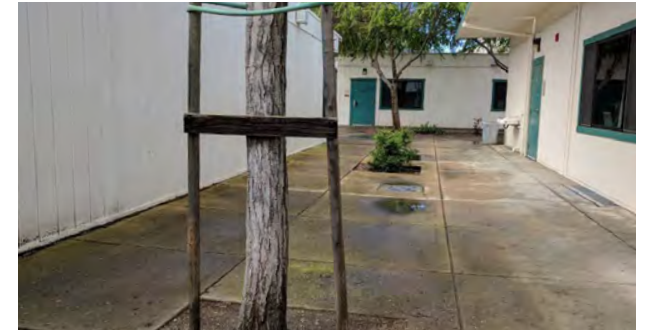
Typical Concrete Paving
