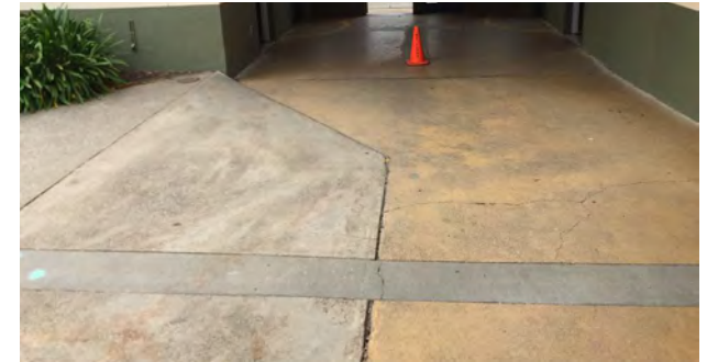
Typical Concrete Paving
