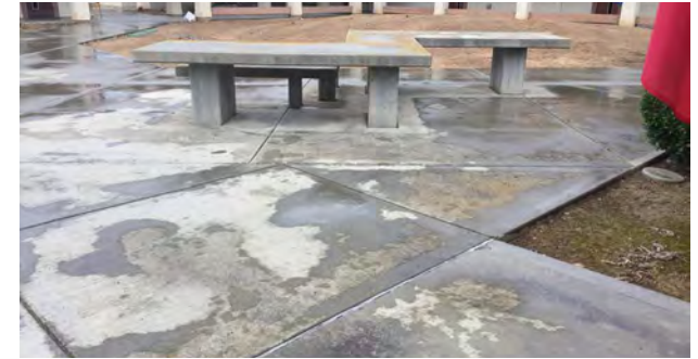
Typical Concrete Paving
