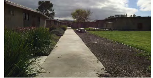
Typical Concrete Paving
