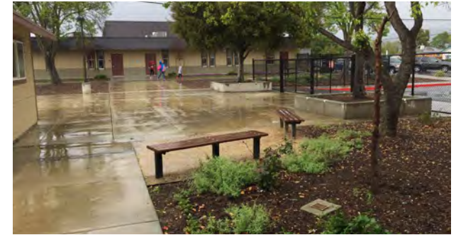
Typical Concrete Paving
