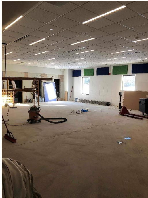
SFMS Cafeteria addition
