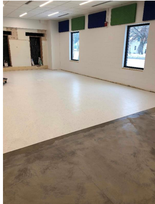
SFMS Cafeteria addition flooring
