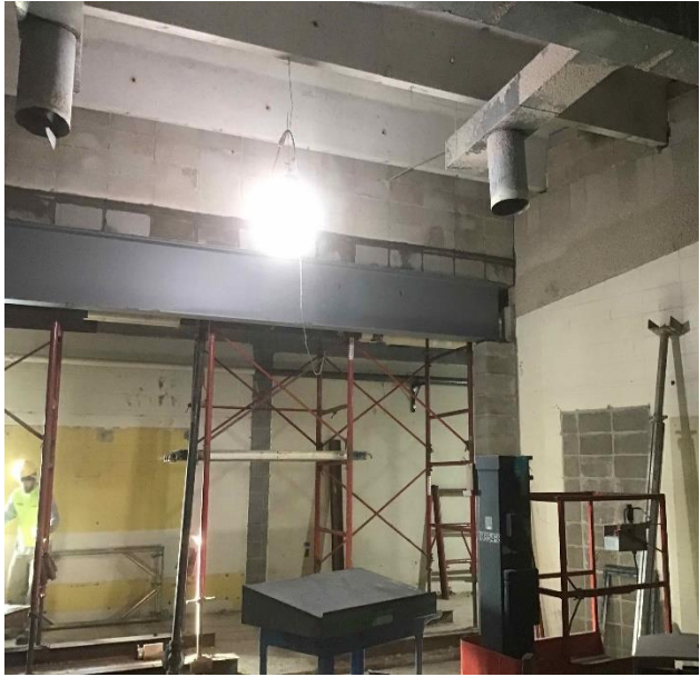
SFHS Band/Choir I beam placement
