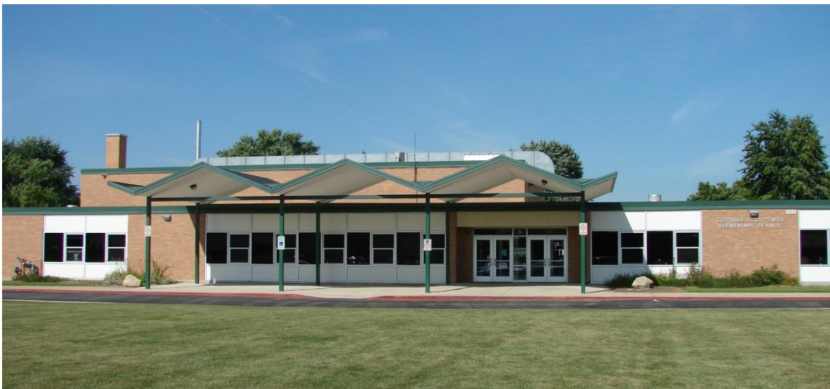
Gertrude Scott Smith Elementary School 1332 Robinwood Drive, Aurora Constructed 1963
