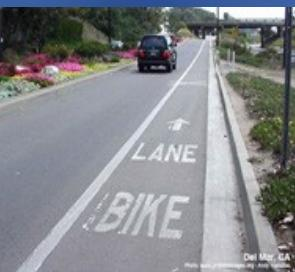
This second type of bike lane is known as a Class II or **Striped Bike Lane**. **Striped bike lanes** aim to provide a clearer sense of where cyclists should be on the road by creating a defined lane for bikes. Usually, these lanes are striped with white paint and are located on the far right side of the road.
