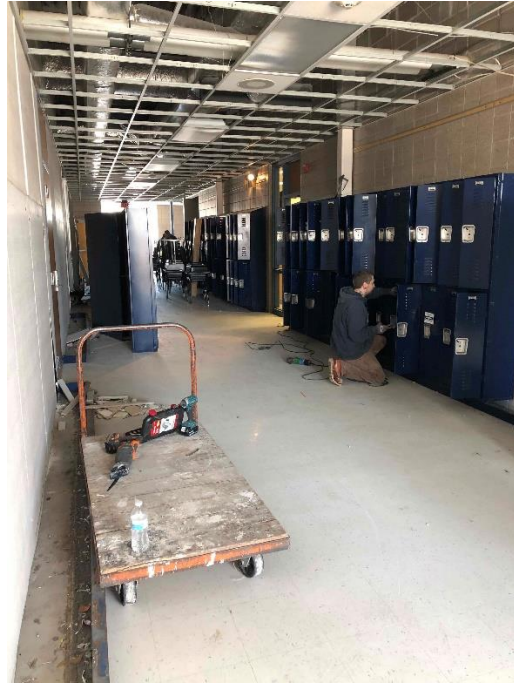
SFMS Locker and Ceiling Demo
