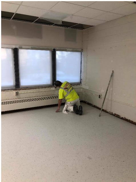
SFMS Classroom Painting
