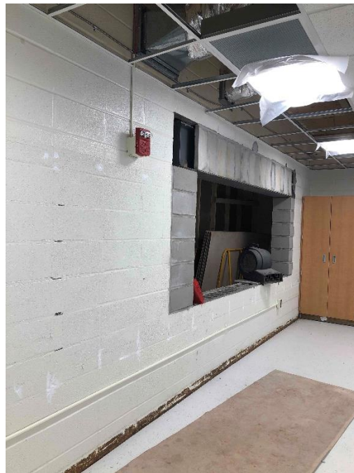
SFMS Classroom Window Block Install
