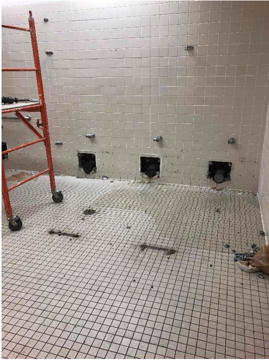
SFMS Bathroom Demo
