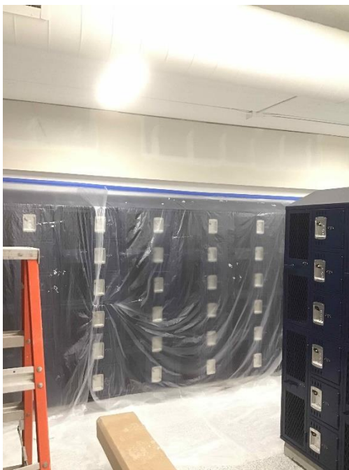
SFHS locker room paint prep
