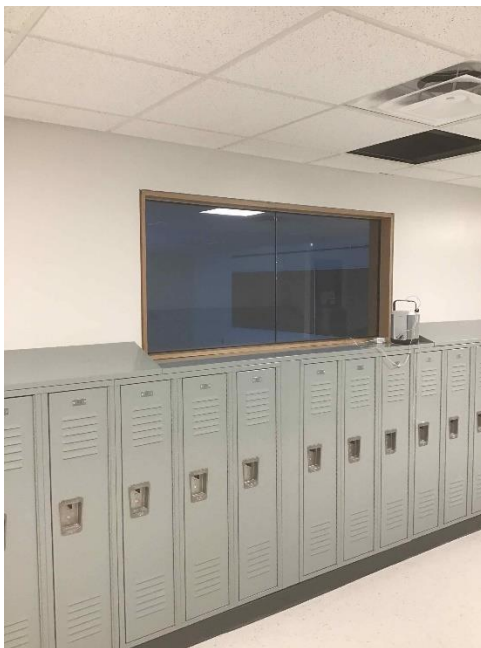
SFES New Addition Windows Installed
