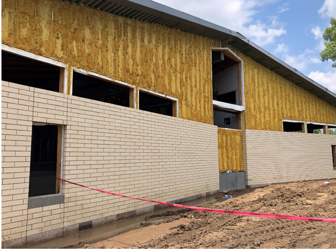
East side brick & West side framing.
