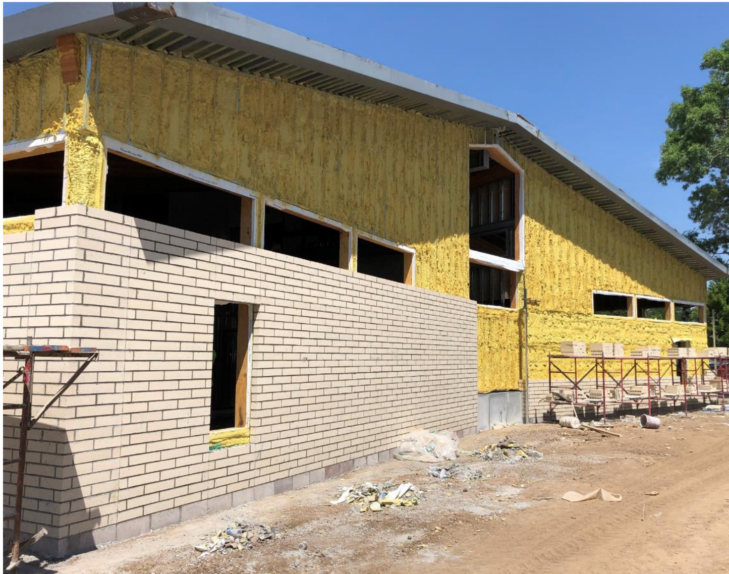
Brick installation on East wing.
