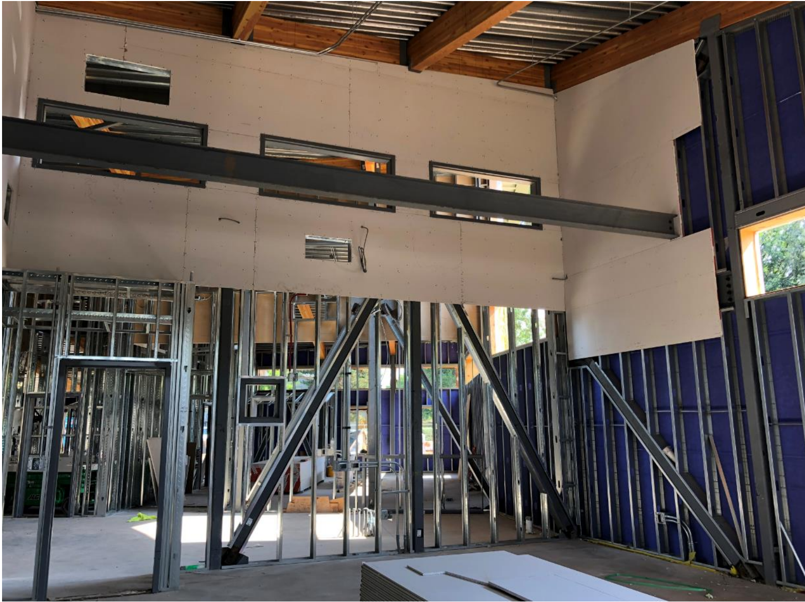
Drywall being installed in classrooms.
