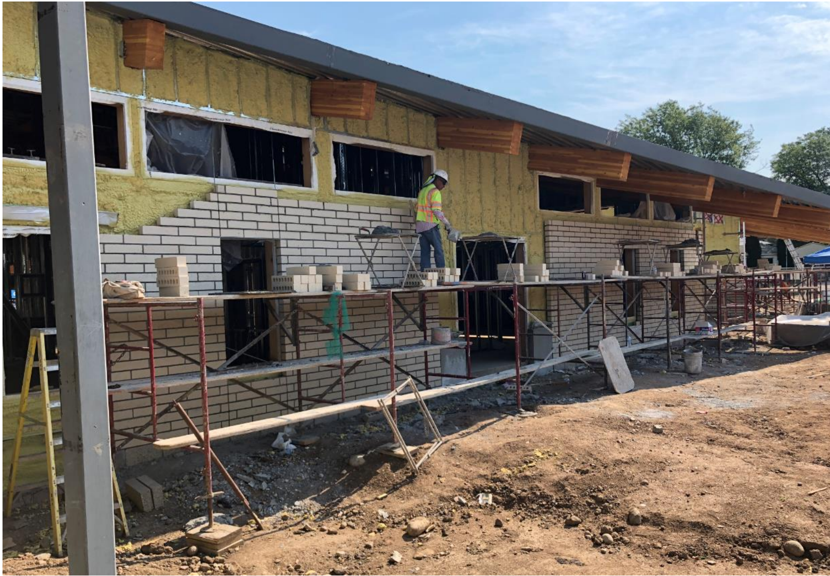
Brick being installed on East wing.
