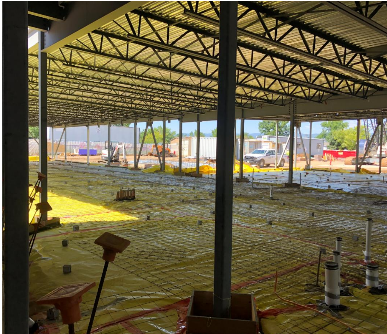
Almost ready to pour slab in Central body.
