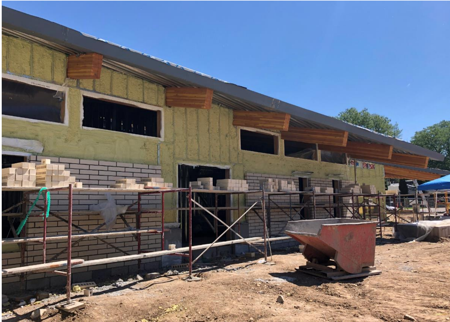
Brick being installed on East wing.
