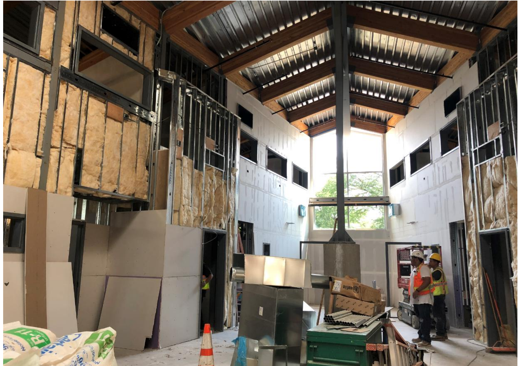
Insulation & Drywall in East wing.
