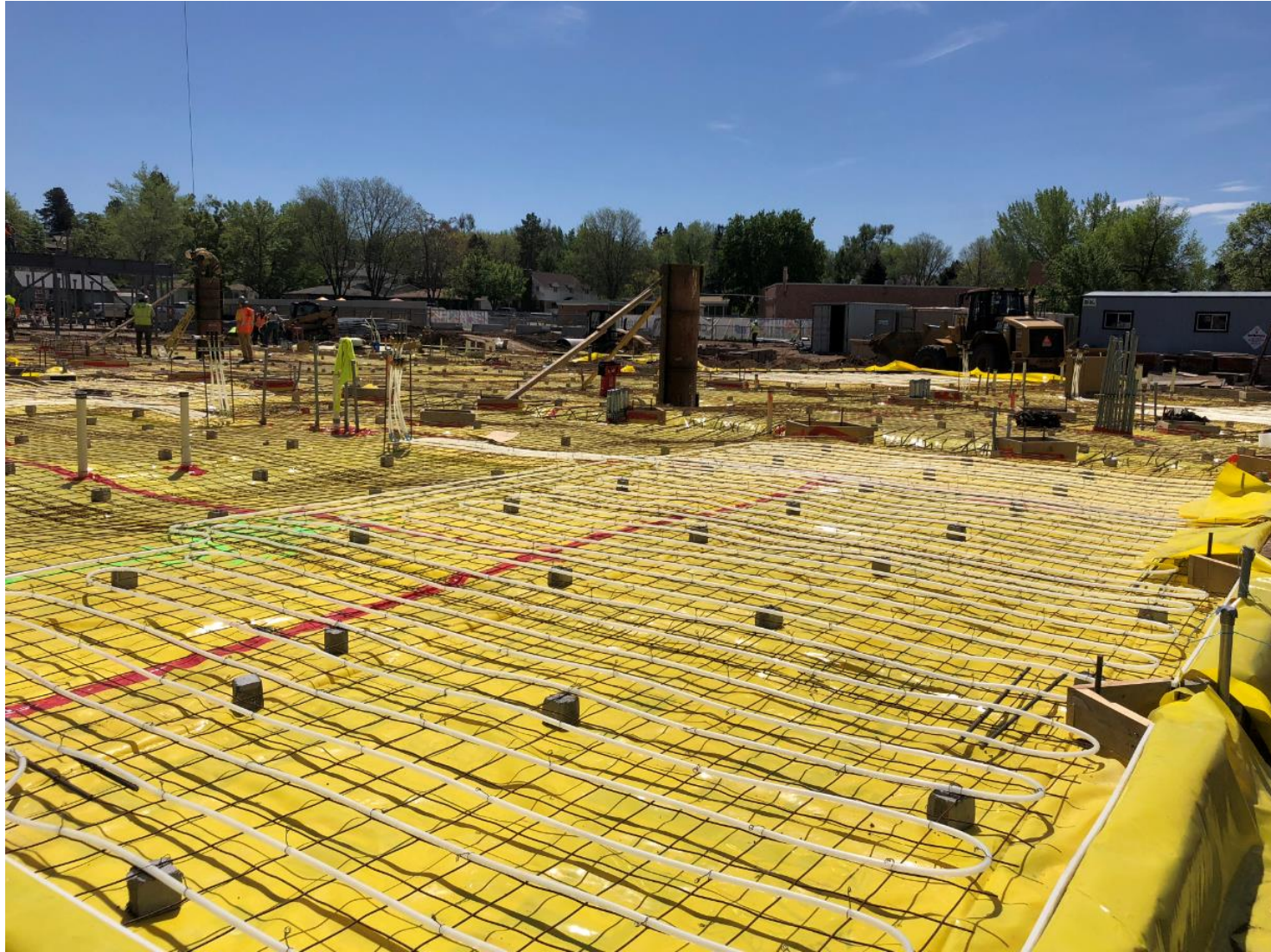
Vapor barrier and radiant heating installed on East wing.
