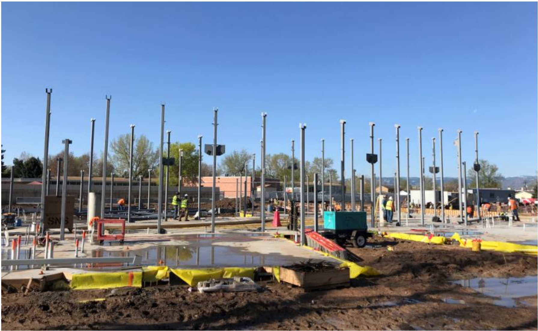
East wing with steel columns and floor slab.
