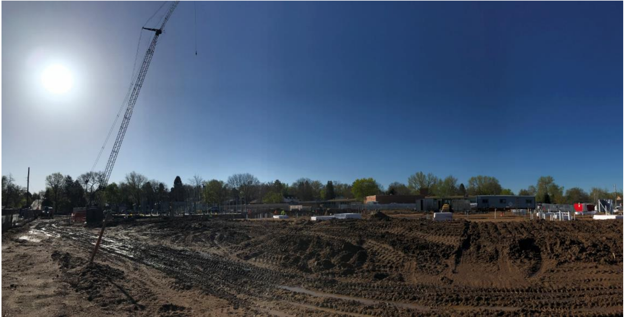
Looking South across entire building footprint.
