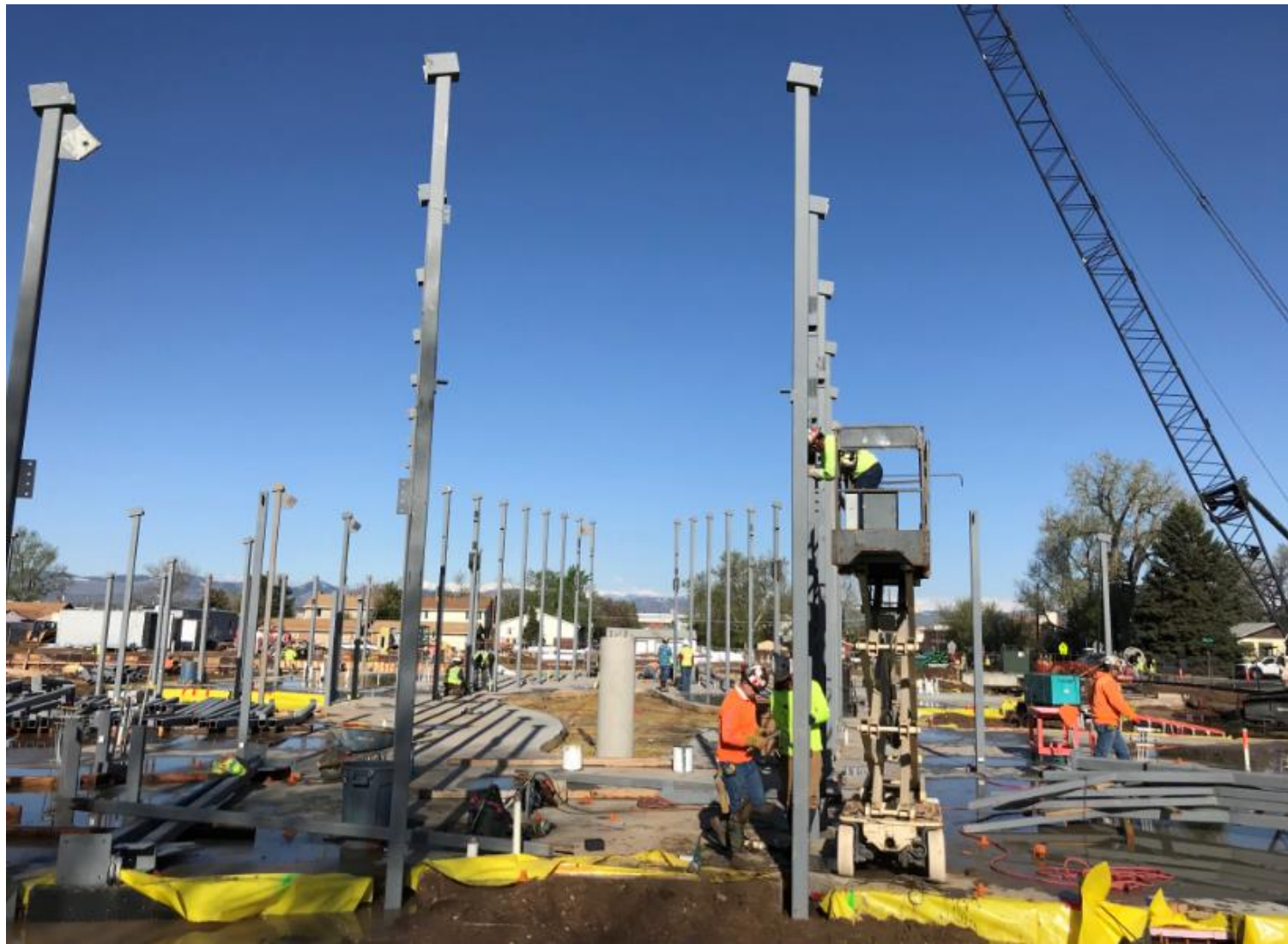
Looking West across building, steel columns installed.
