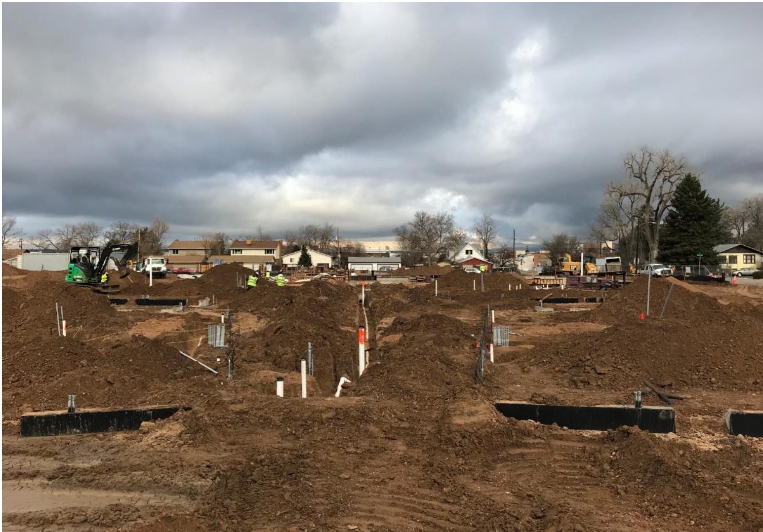
Looking West – backfilled with utility stub-ups.
