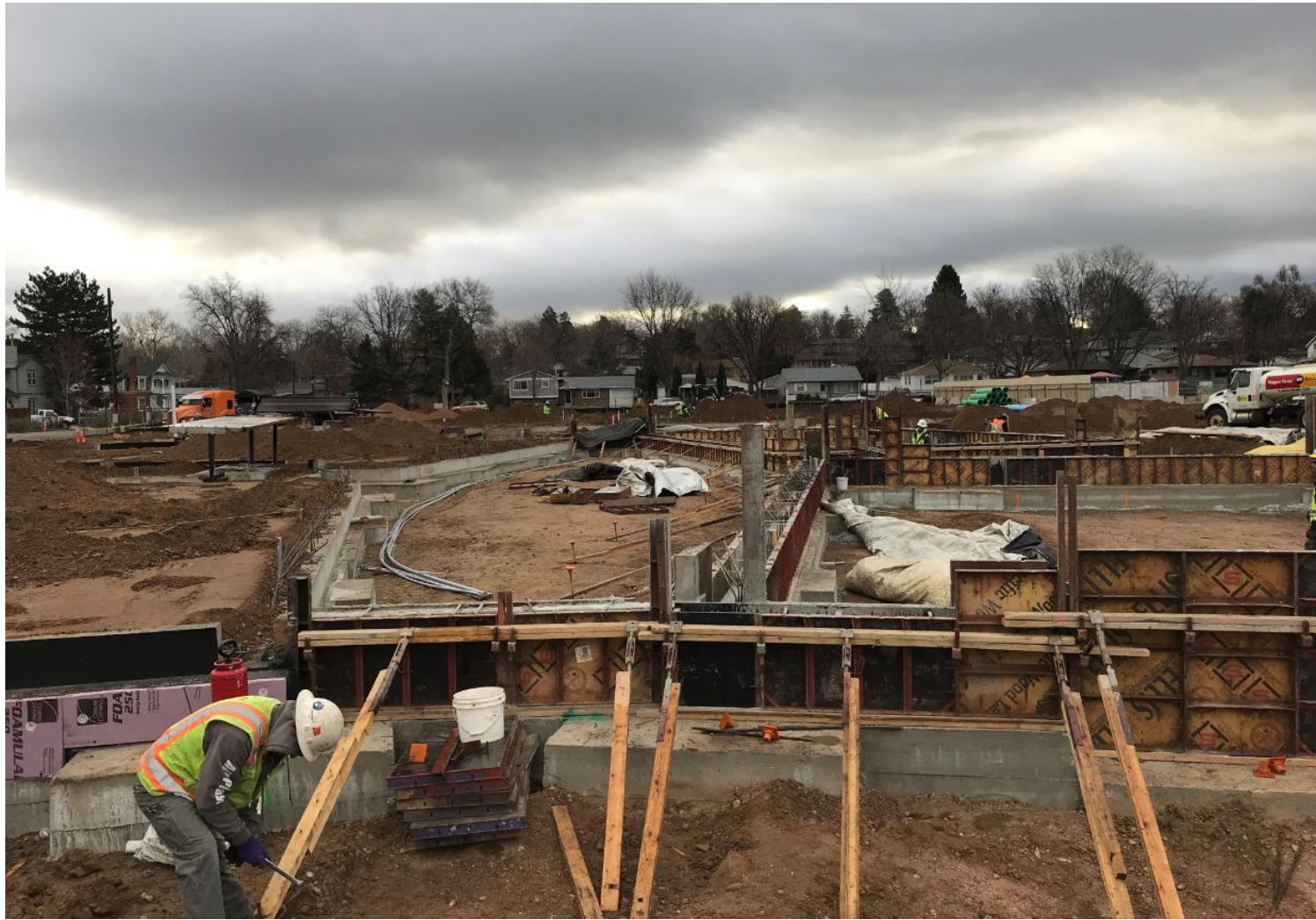
Looking East – North stem walls poured, South are formed.
