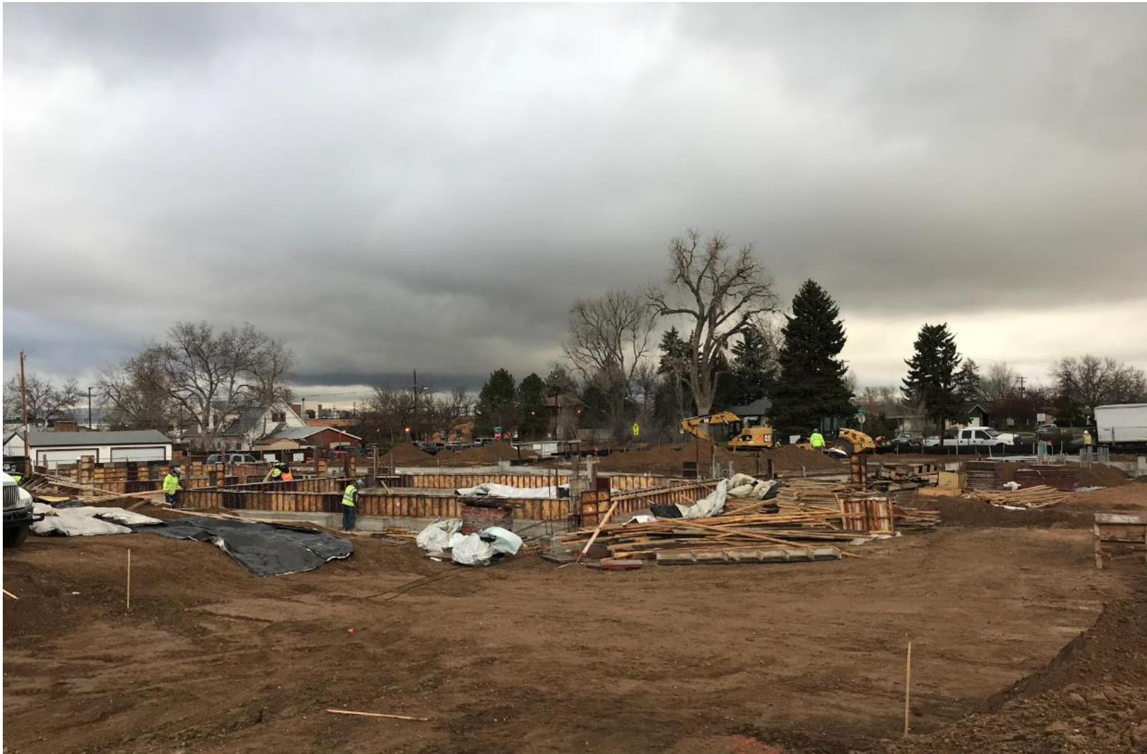
West wing stem walls half poured.
