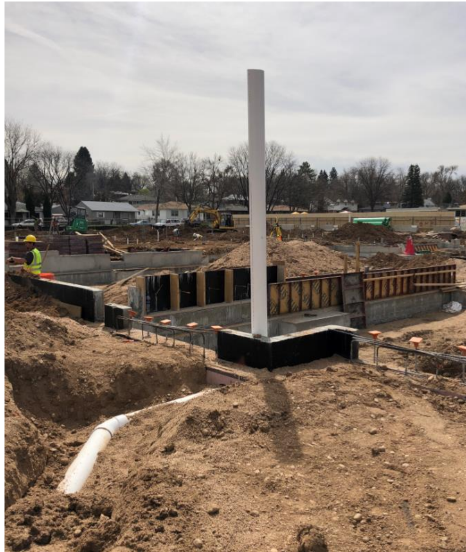
Roof drain to underground storm drain.
