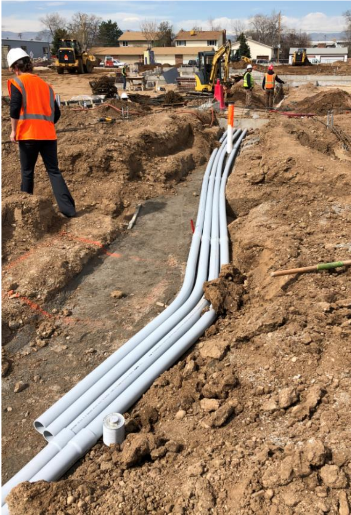
Underground IT conduit from MDF to Storage Rooms (left). IT conduit coming up to Teaching Wall (right).
