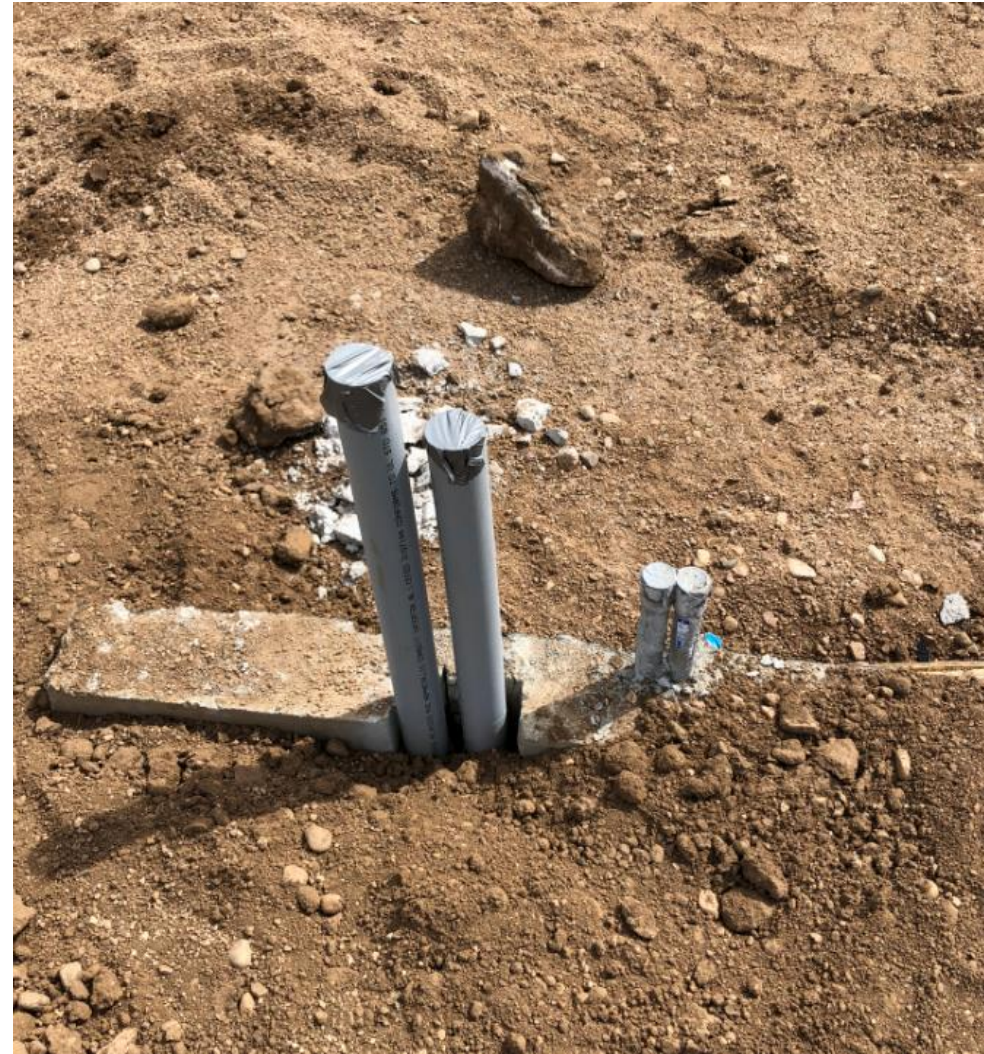
Underground IT conduit from MDF to Storage Rooms (left). IT conduit coming up to Teaching Wall (right).
