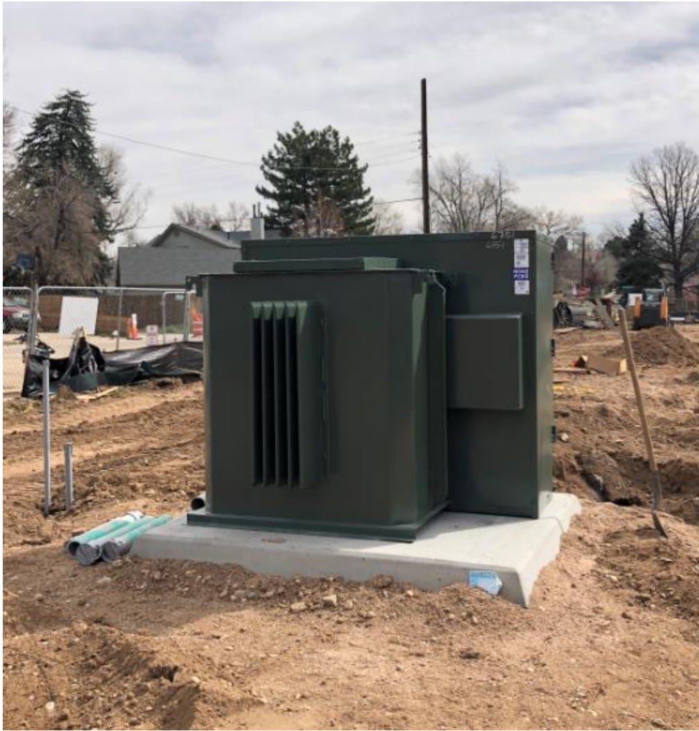
Transformer set (left). Conduit to Electrical room (right).
