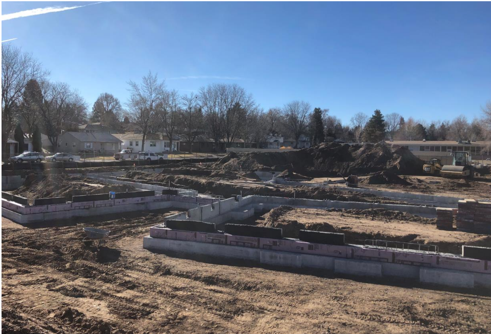
East wing with stem wall poured.
