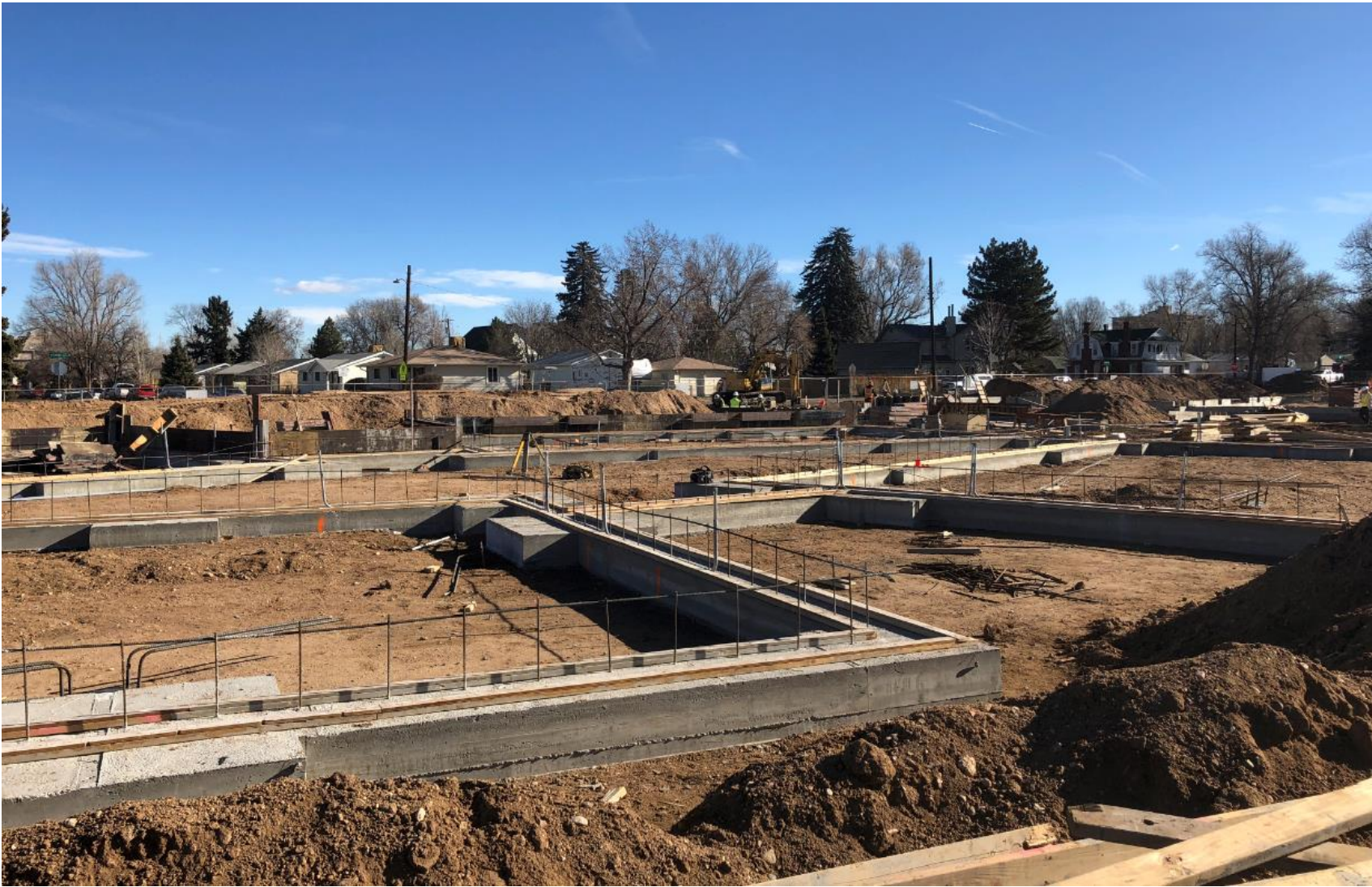
West wing stub-ups and stem wall rebar.
