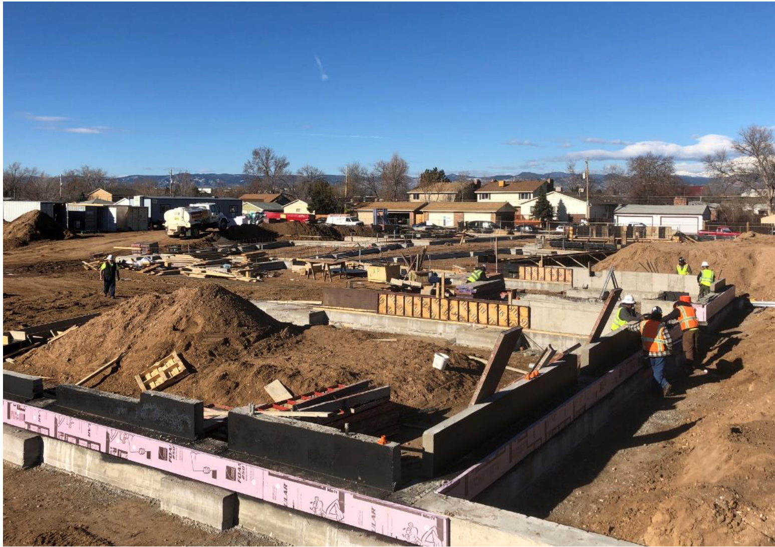
North central section, closeup of insulation, dampproofing and IT conduit.
