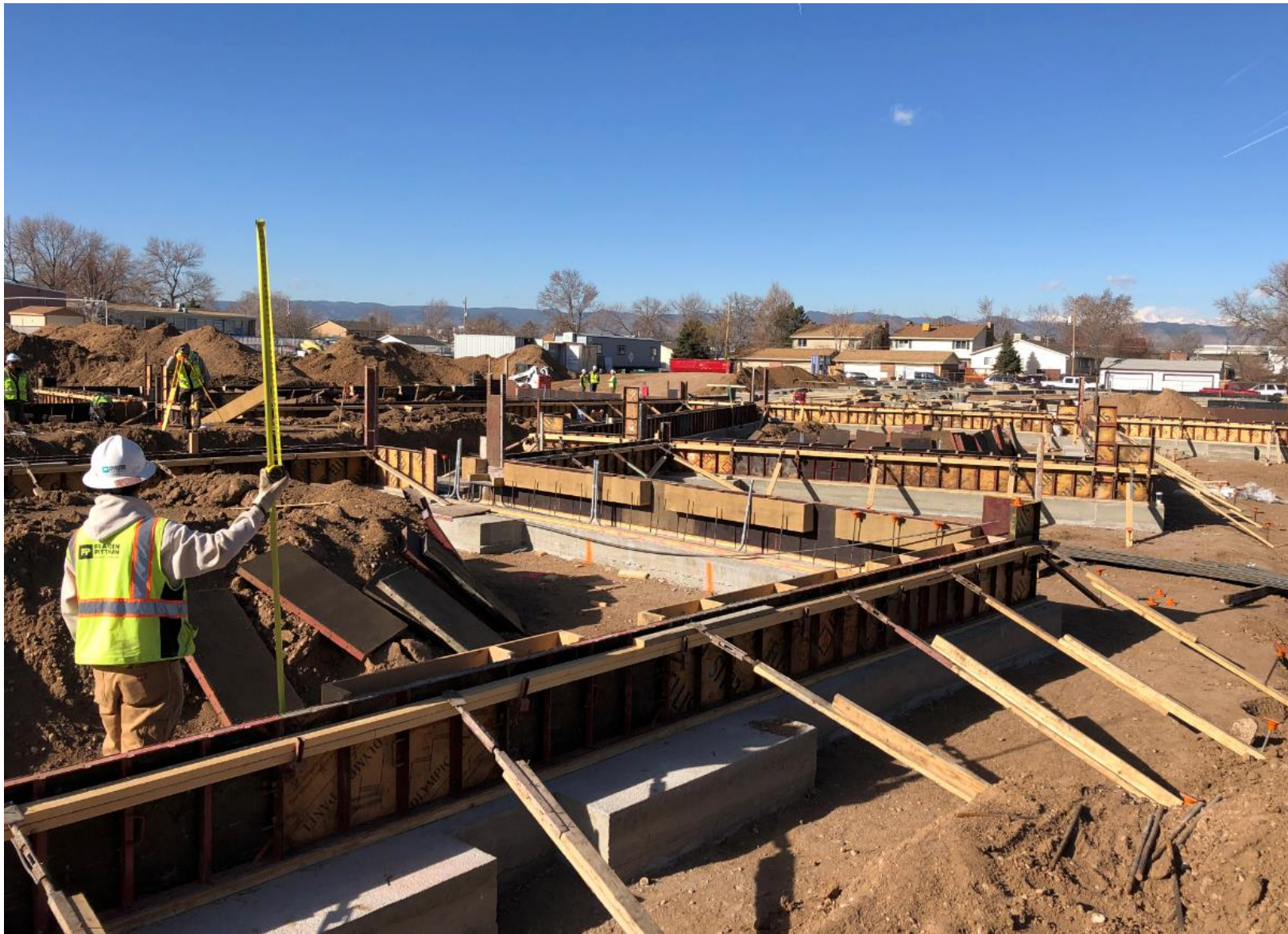
Using surveying equipment to perform quality control on stem wall forms.
