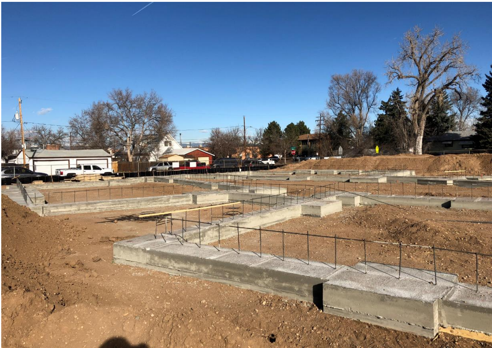
Stem wall rebar at West wing.
