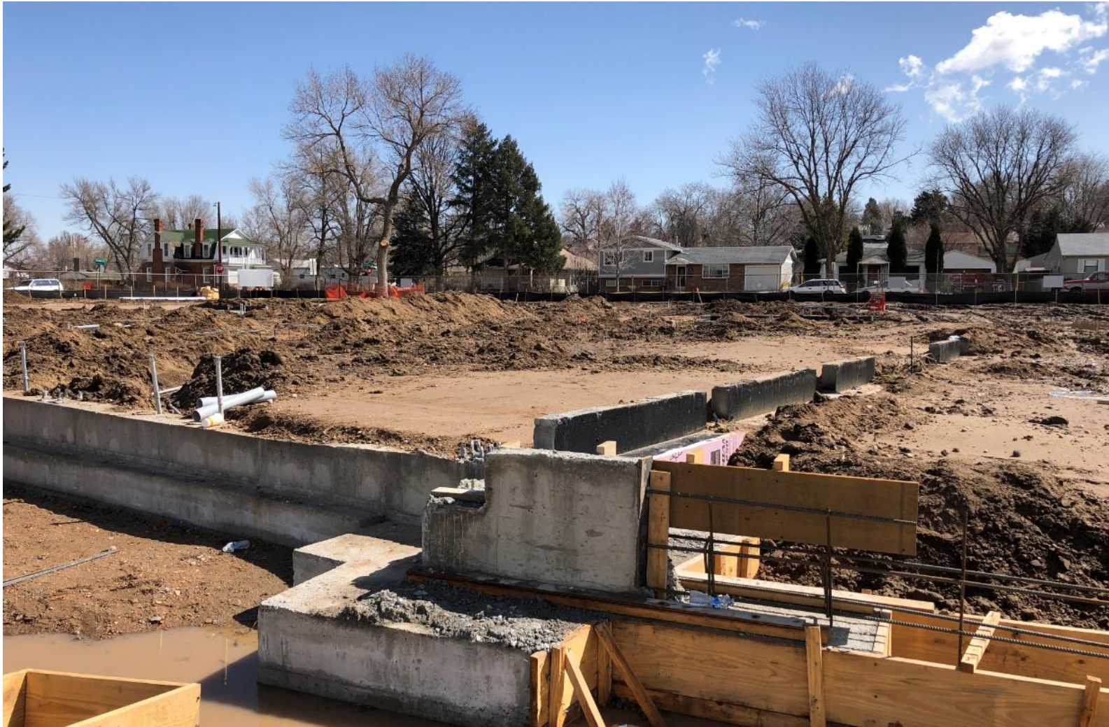
East wing backfilled.
