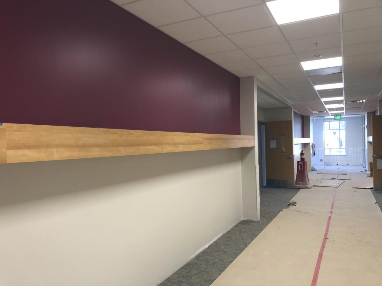
Kindergarten Wing – Paint and flooring newly complete.
