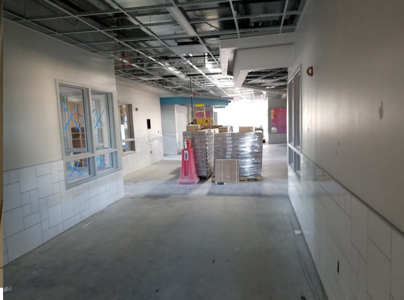
South Classroom Wing (upper level) – Carpet to be installed soon.
