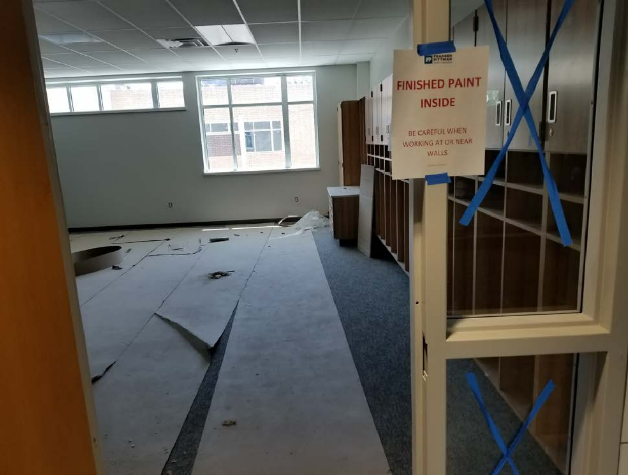
North Classroom Wing (upper level) – Classroom; Ceiling tile newly installed.
