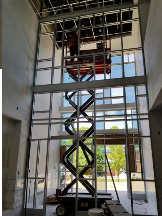
Grand Hall – North Facing View; Windows and ceiling being installed.
