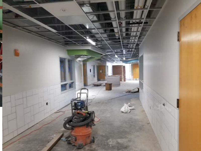
North Classroom Wing (L1) – Flooring to be installed soon.
