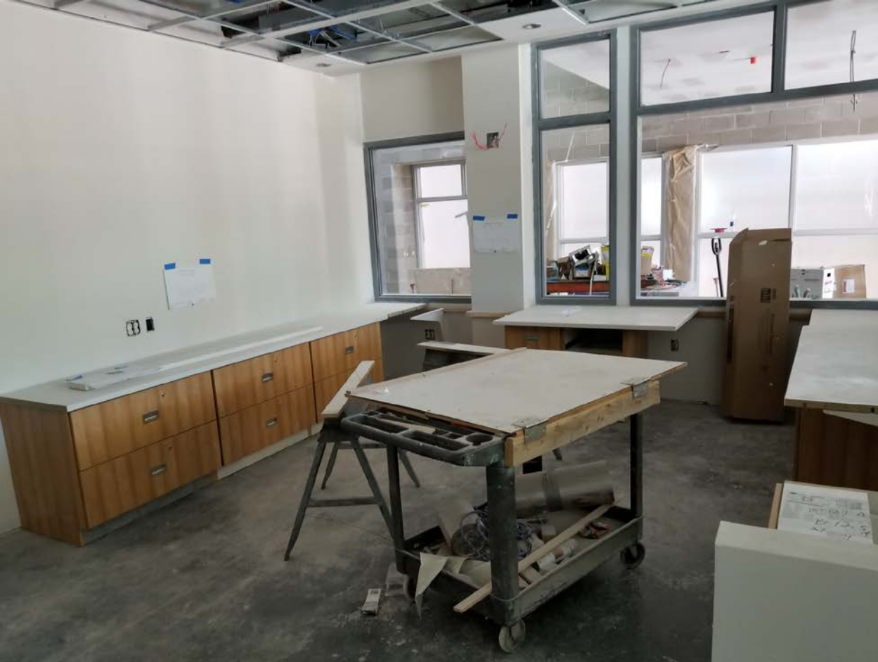
Reception Area – Cabinets being installed.
