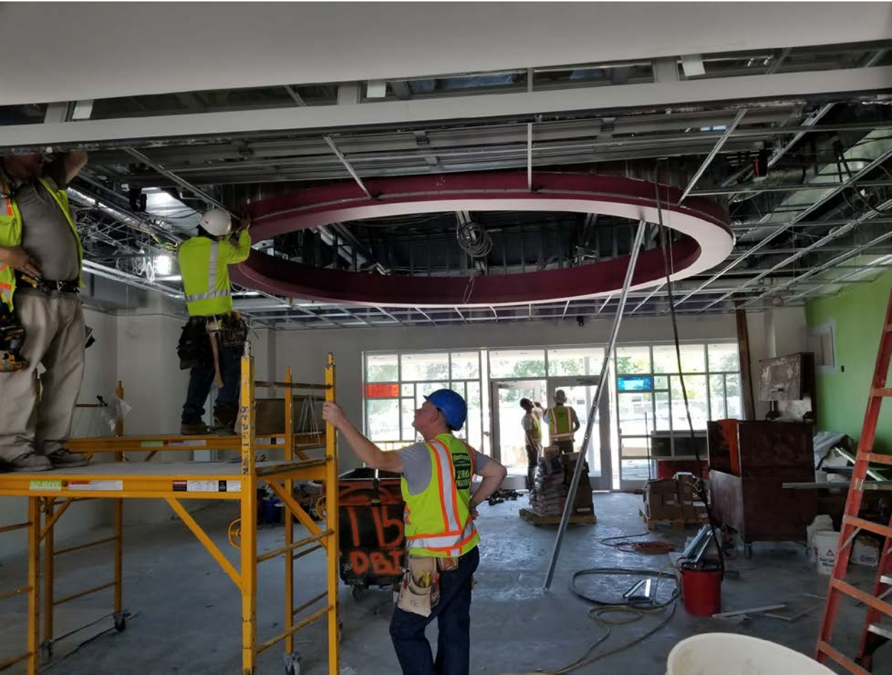
Cafeteria – Painting, HVAC and electrical work continues.
