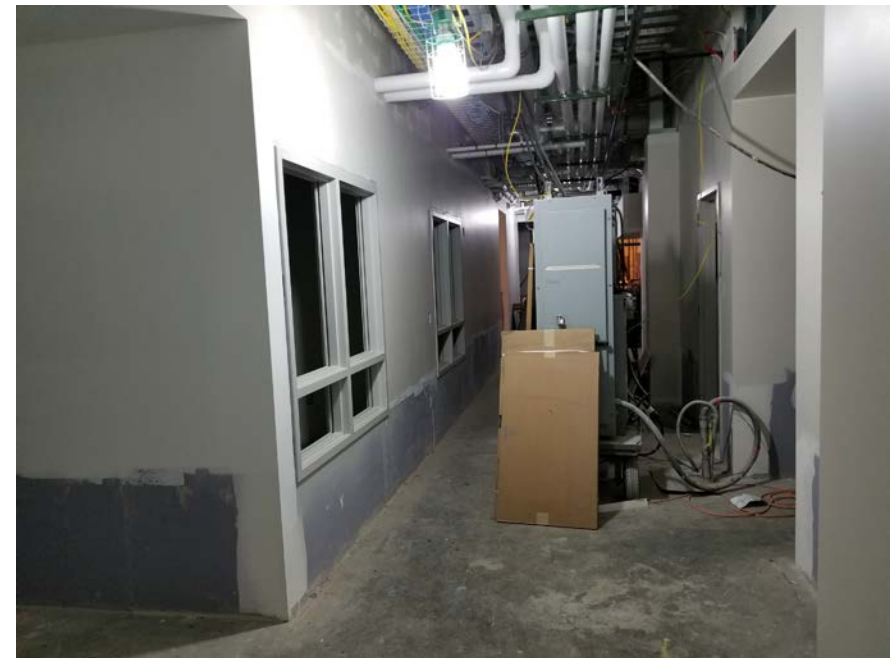
South Classroom Wing (lower level) – Tilework to begin soon.
