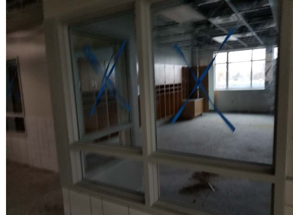
North Classroom Wing (upper level) – Glass in classroom newly installed.
