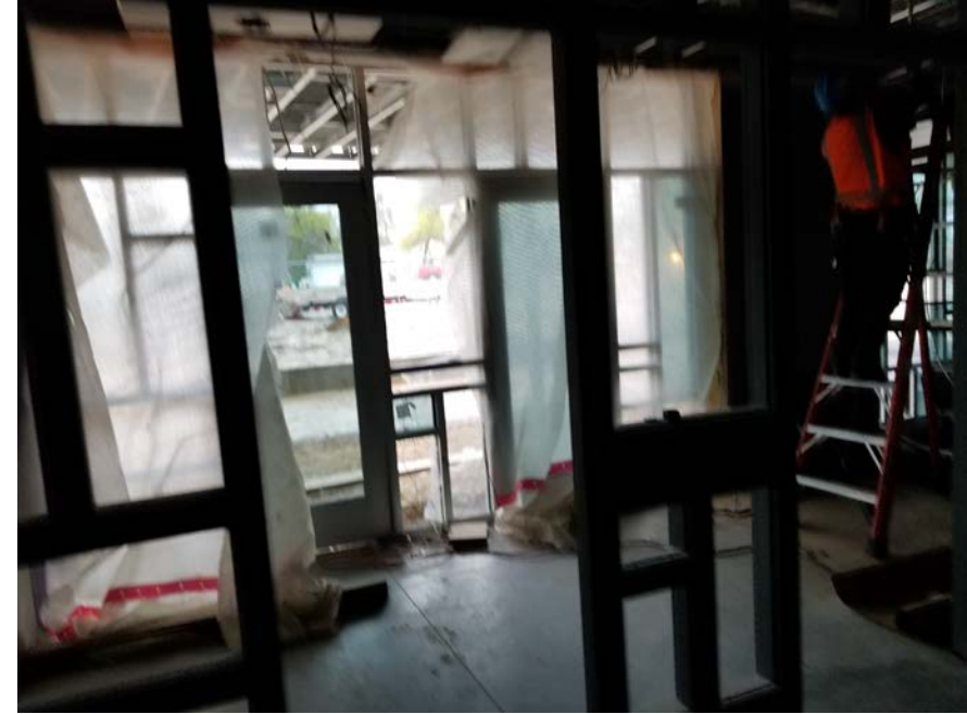
Main Entrance – Entry doors newly installed.
