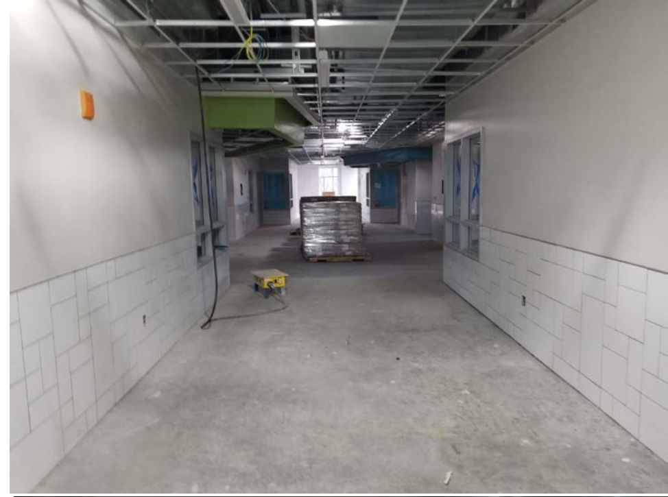
North Classroom Wing (upper level) – Light fixtures newly installed and wall tile complete.
