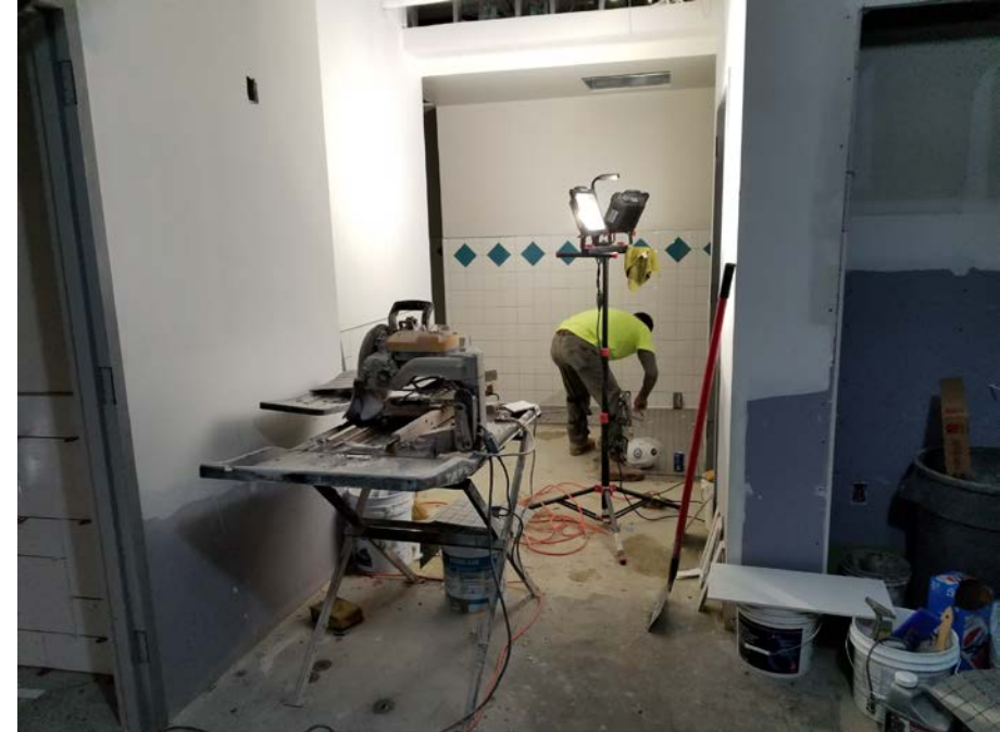
North Classroom Wing (lower level) – Restrooms; Floor tile install continues.
