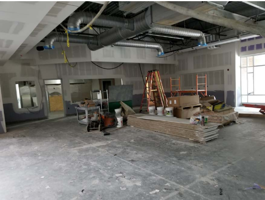
Cafeteria – HVAC and electrical work continues. Painting to begin soon.
