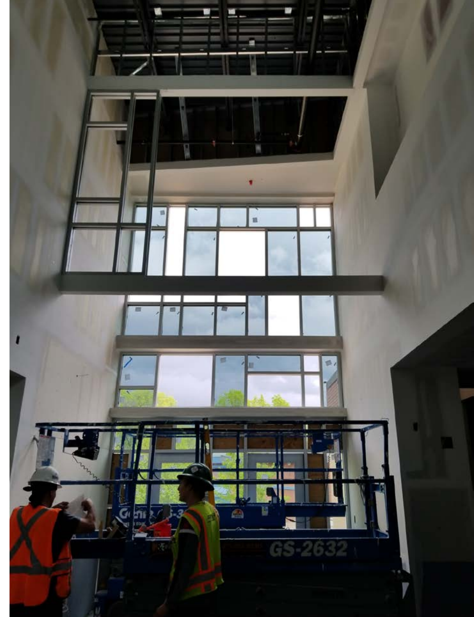
Grand Hall – North Entrance; Framing and glass install.
