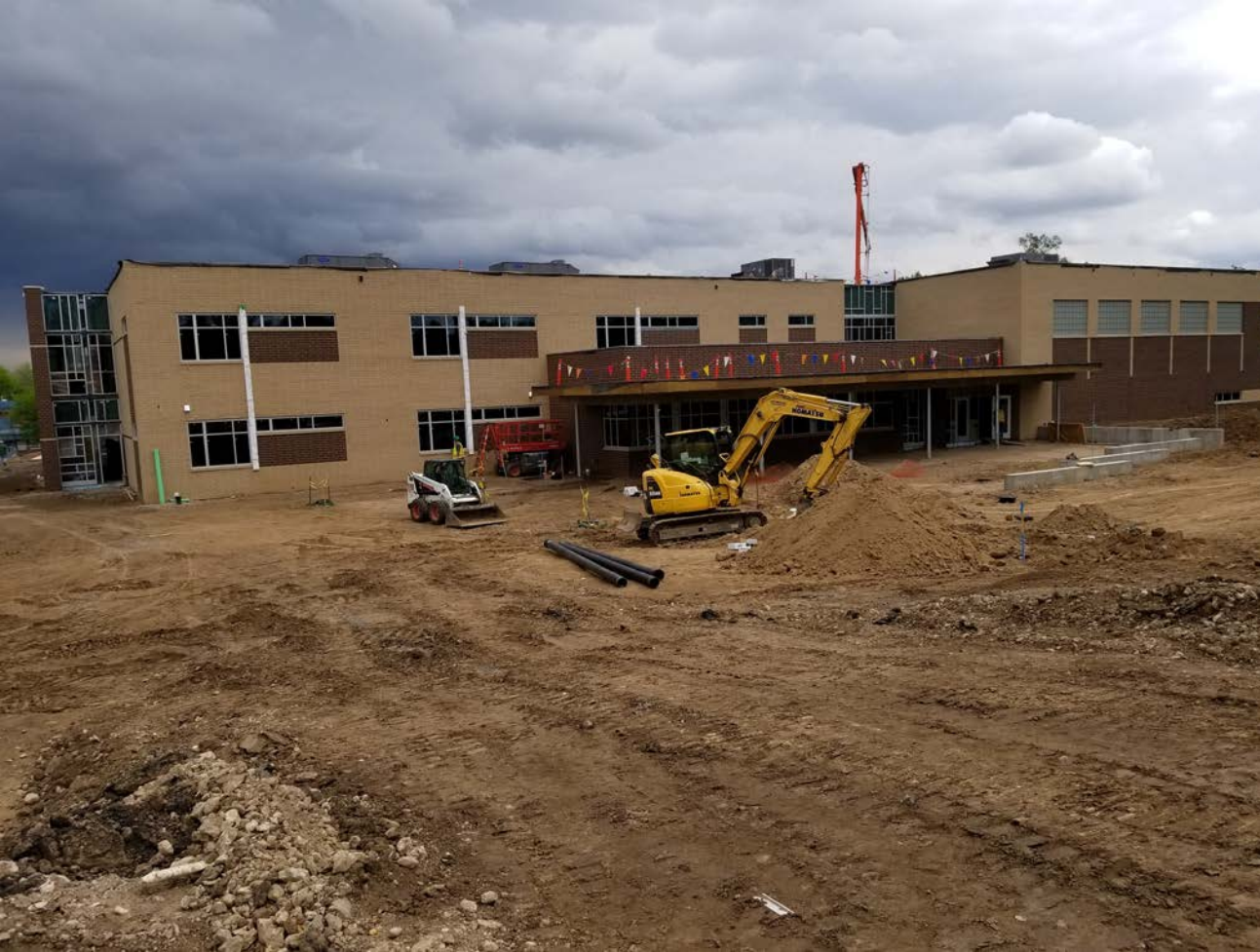
South Elevation – Main Entrance; Sitework continues.
