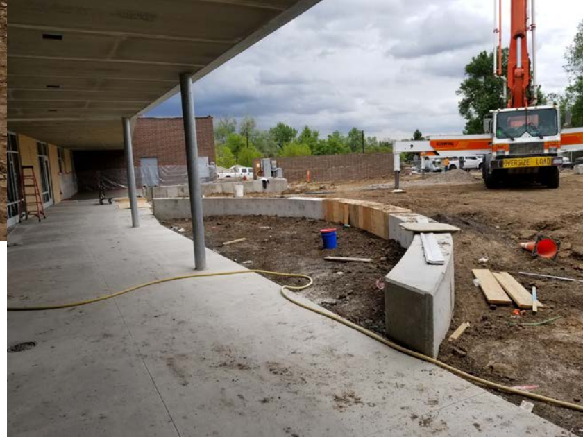
East Elevation – Sitework continues.
