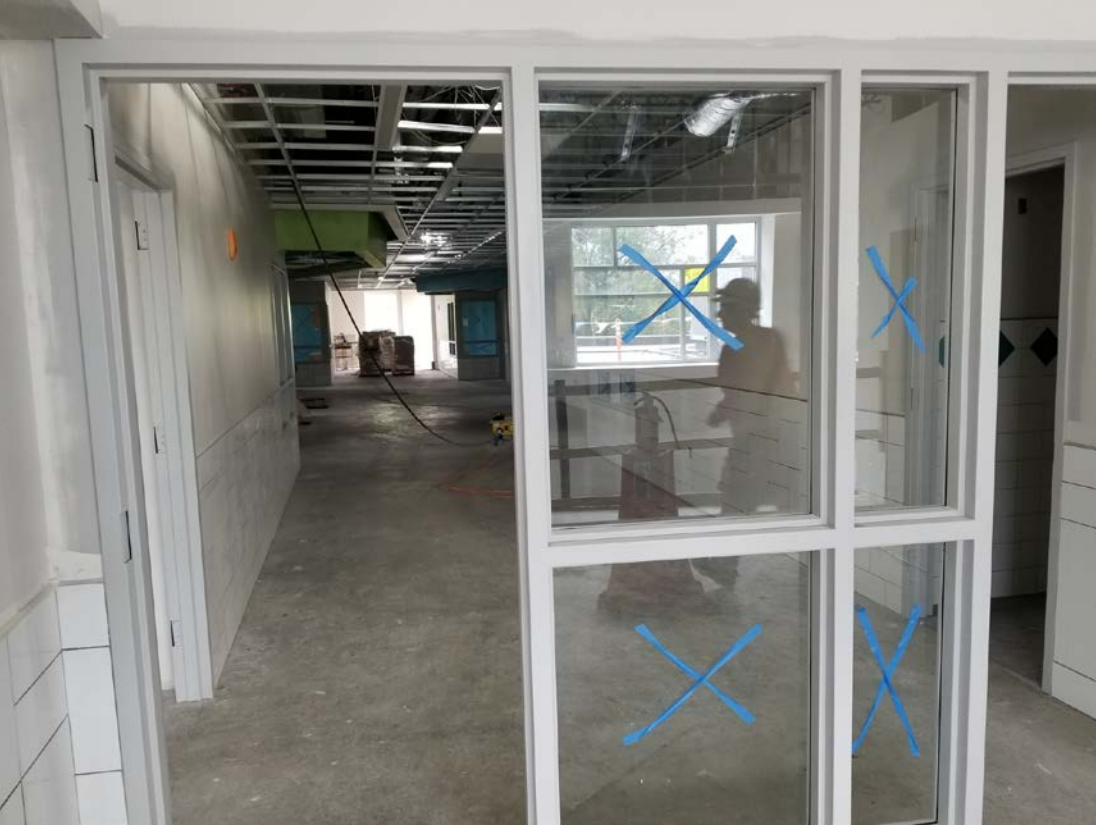
North Classroom Wing (upper level) – Glass recently installed.
