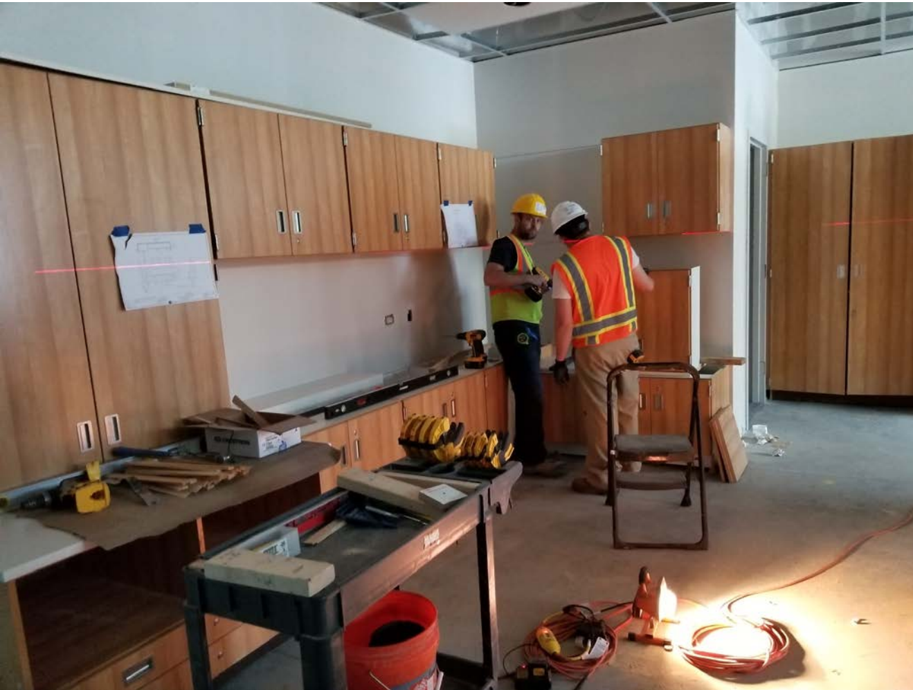
South Classroom Wing (L1) – Classroom; Cabinets being installed.
