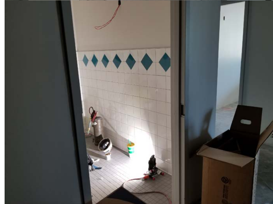
South Classroom Wing (lower level) – Teacher Restroom; Tilework in progress.
