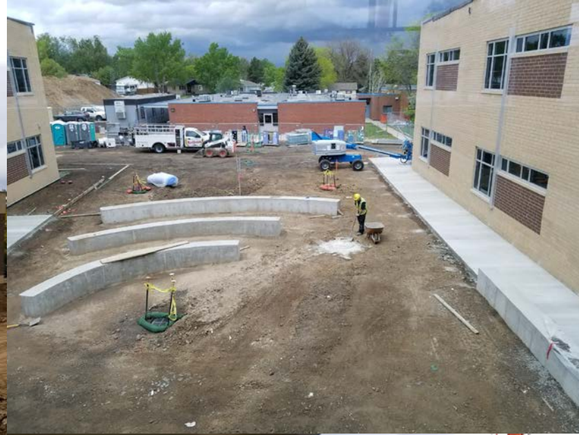
West Elevation – Plaza Between Classrooms; Sitework continues, walkways newly poured.
