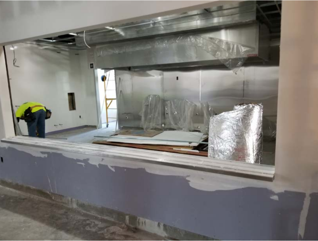
Cafeteria – Kitchen equipment infrastructure being installed.
