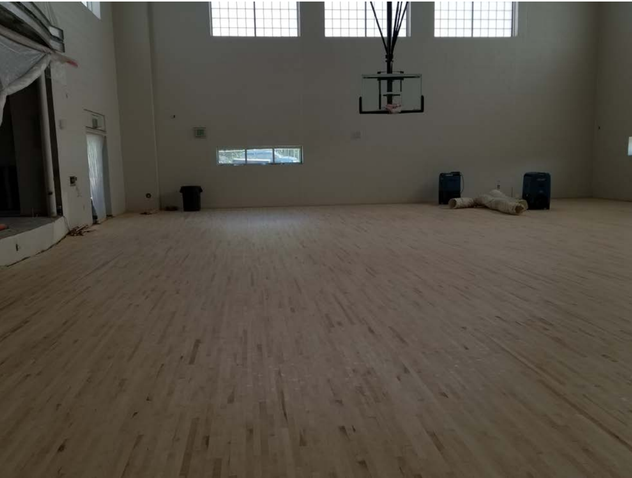
Gym – Flooring newly installed.
