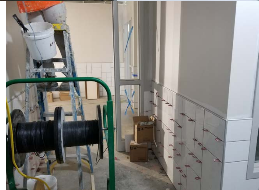
South Classroom Wing (L1) – SPED Area; Tilework in progress.
