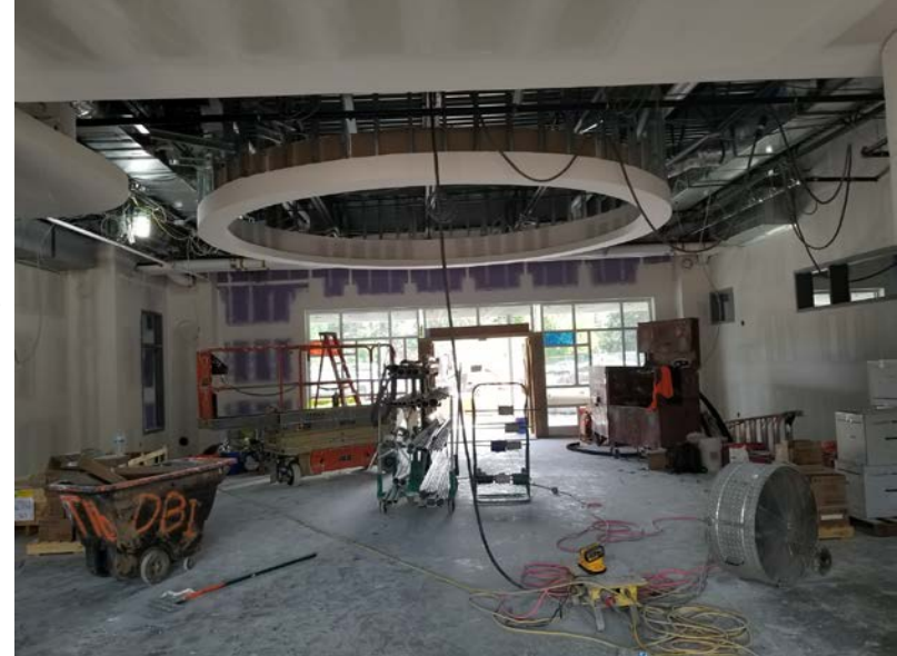
Learning Commons – Mechanical, electrical, and ceiling work continues.
