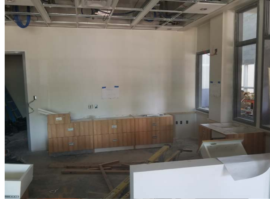
Admin Area – Cabinets being installed.
