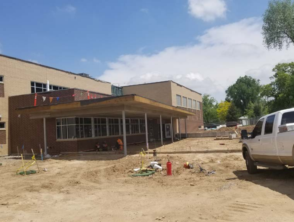
South Elevation – Main Entrance; Sitework continues, concrete to be poured soon.
