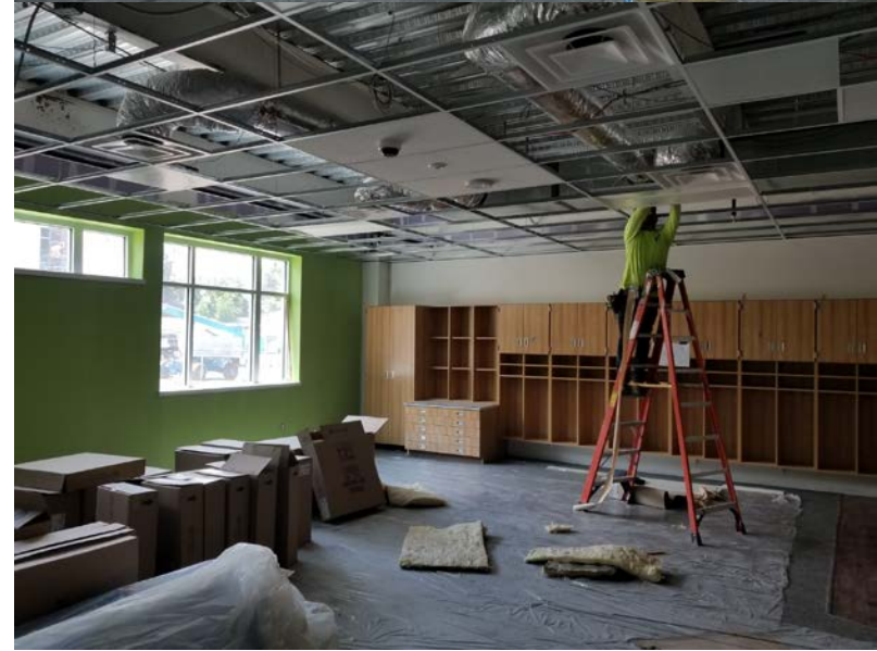
North Classroom Wing (lower level) – Classroom; Ceiling tile being installed.
