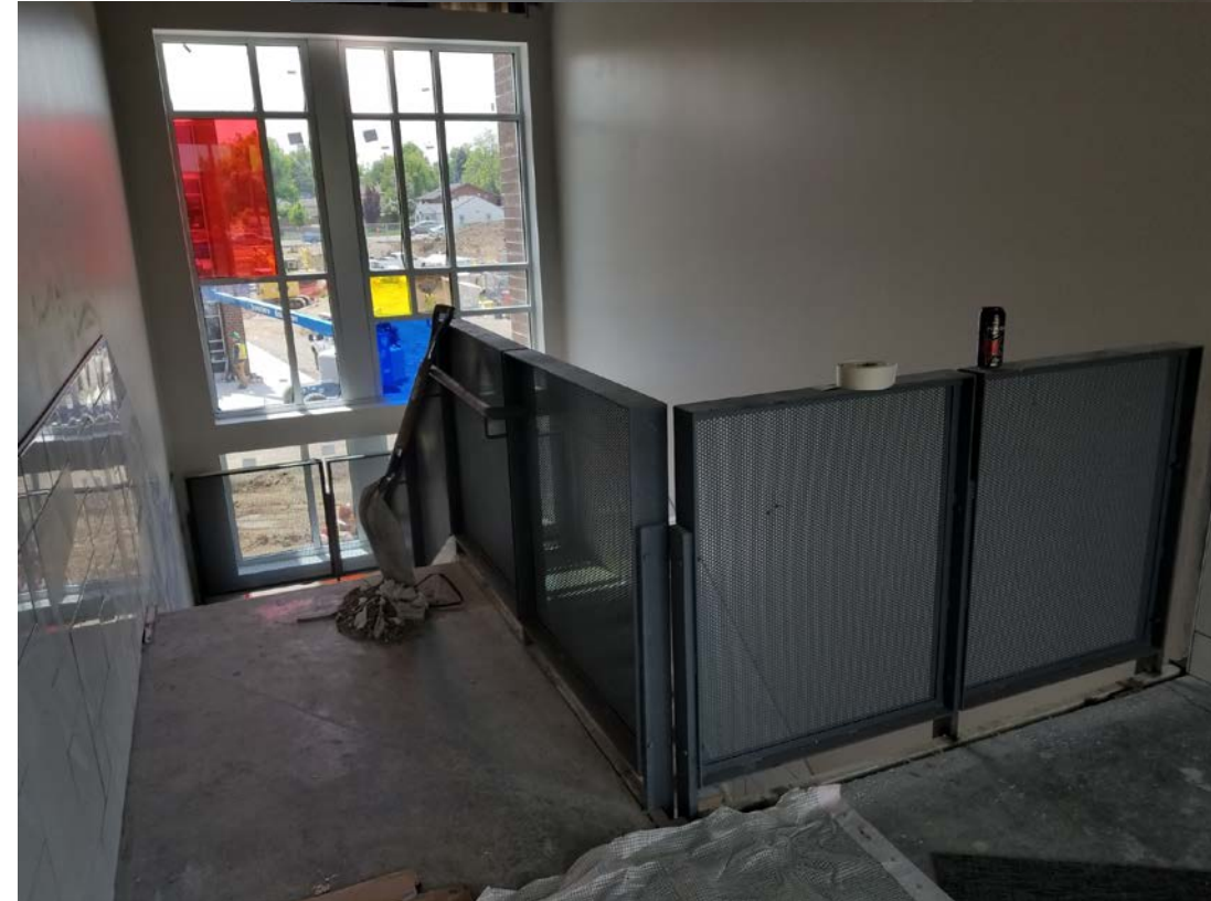
North Classroom Wing (upper level) – Flooring to be installed soon.
