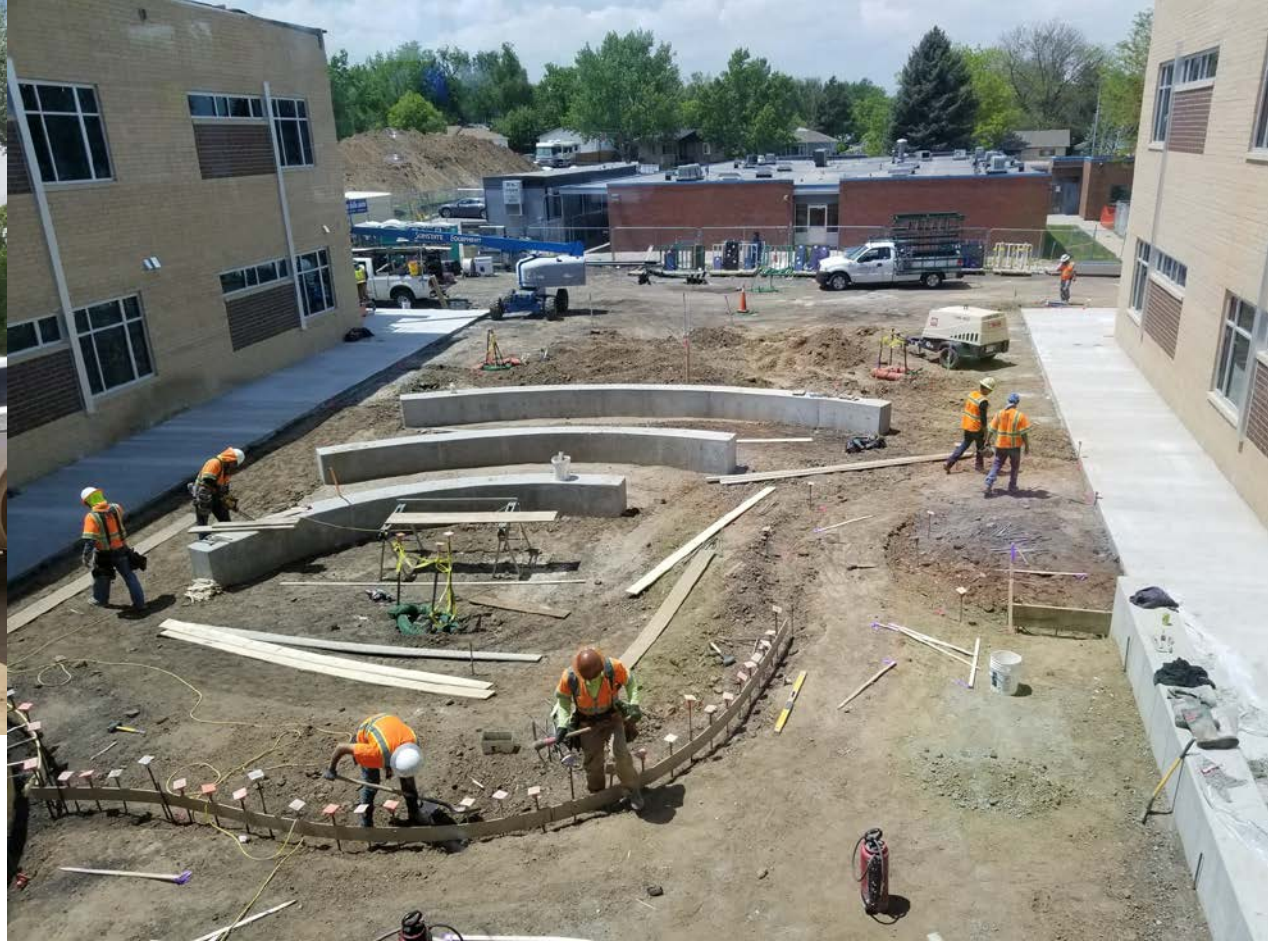
East Elevation – Plaza Between Classroom Wings; Sitework continues, concrete newly poured.
