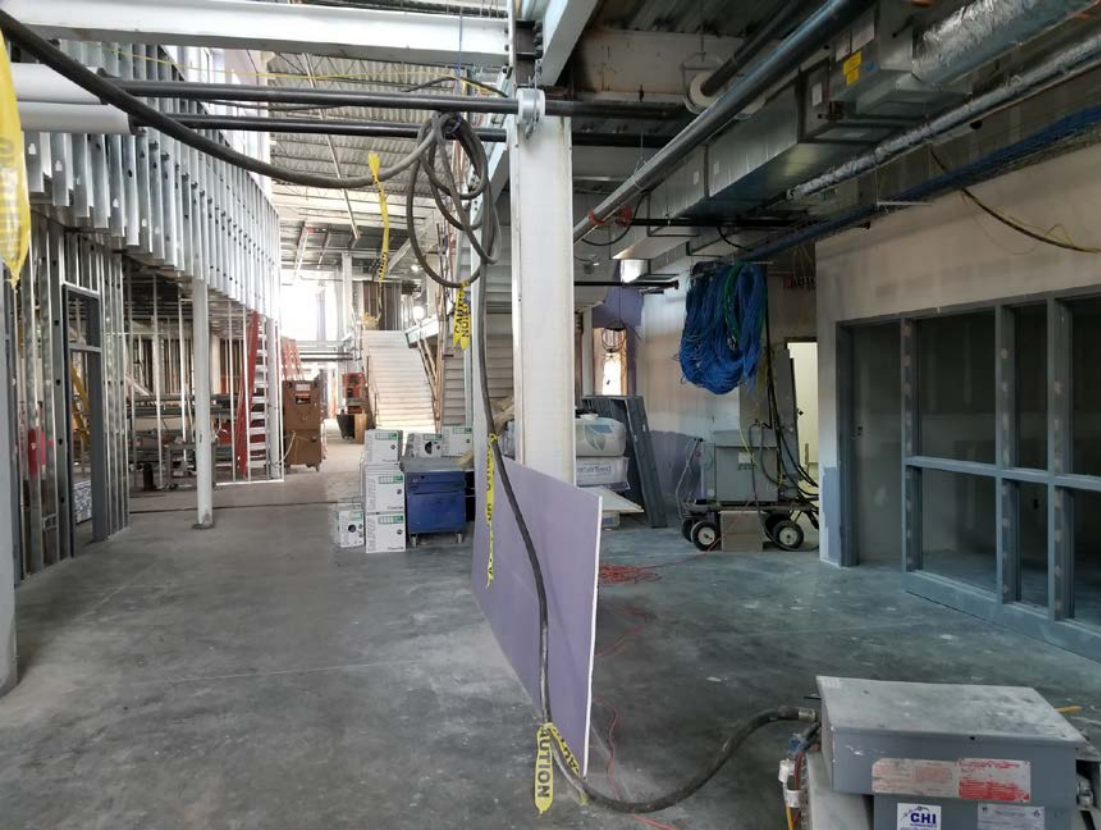
Grand Hall – South Facing View; Framing, mechanical, and drywall install continues
