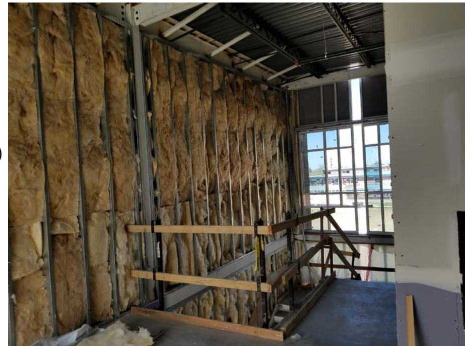
South Classroom Wing (upper level) – Stairwell; Insulation and drywall install.
