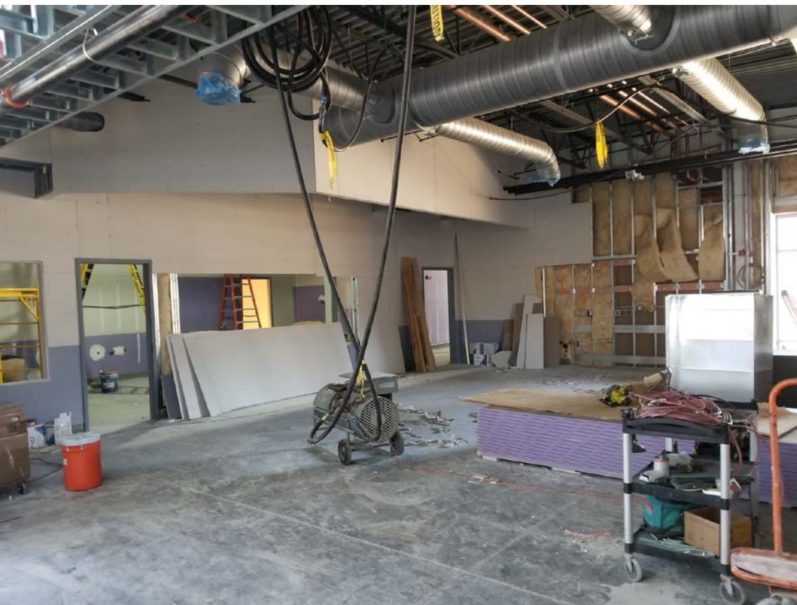
Cafeteria – Drywall and HVAC install continues.
