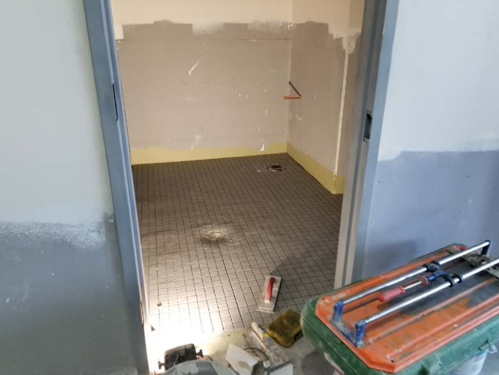
North Classroom Wing (upper level) – Teacher Restroom; Floor tile install.
