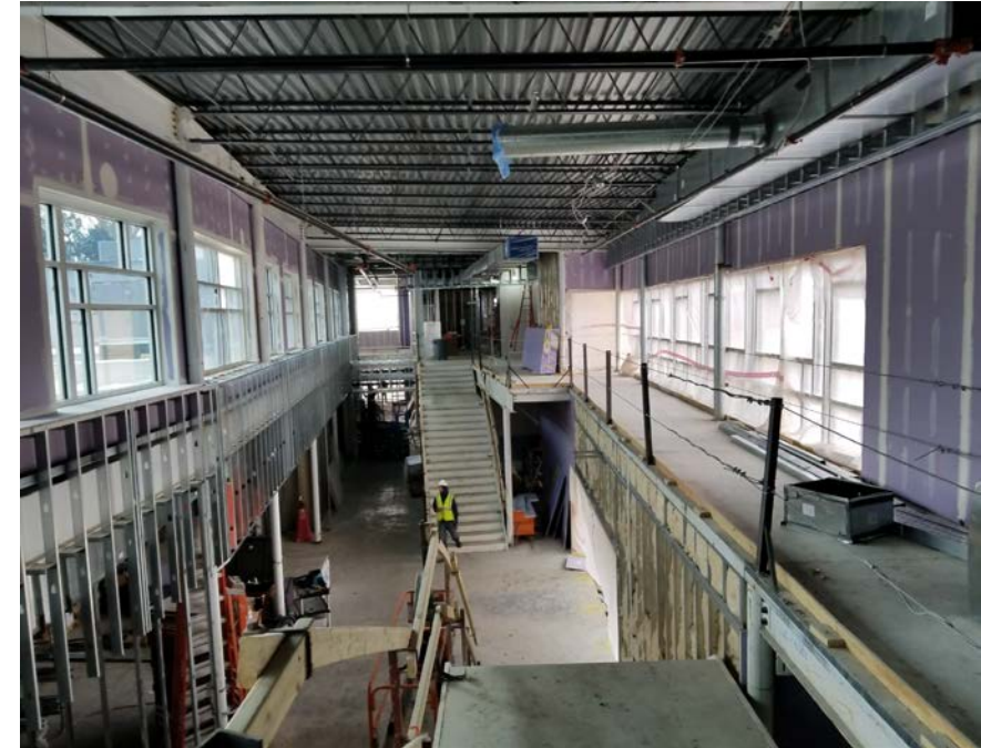
Grand Hall – South Facing View; Framing, mechanical, insulation and drywall install continues
