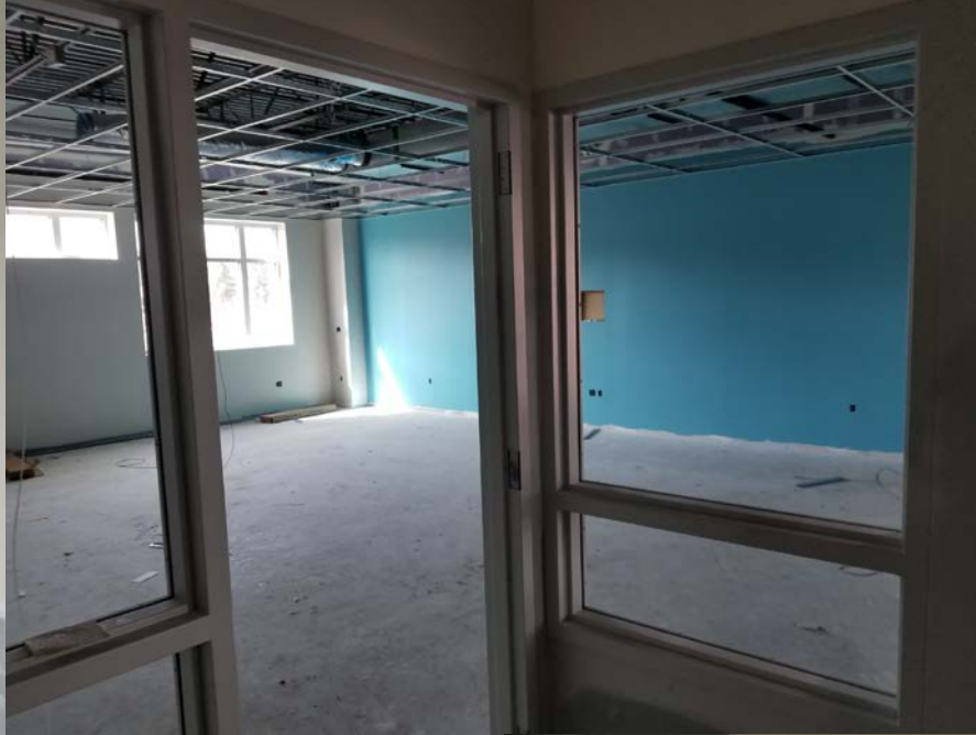
North Classroom Wing (upper level) – Classroom; Painting continues. Ceiling grid being installed
