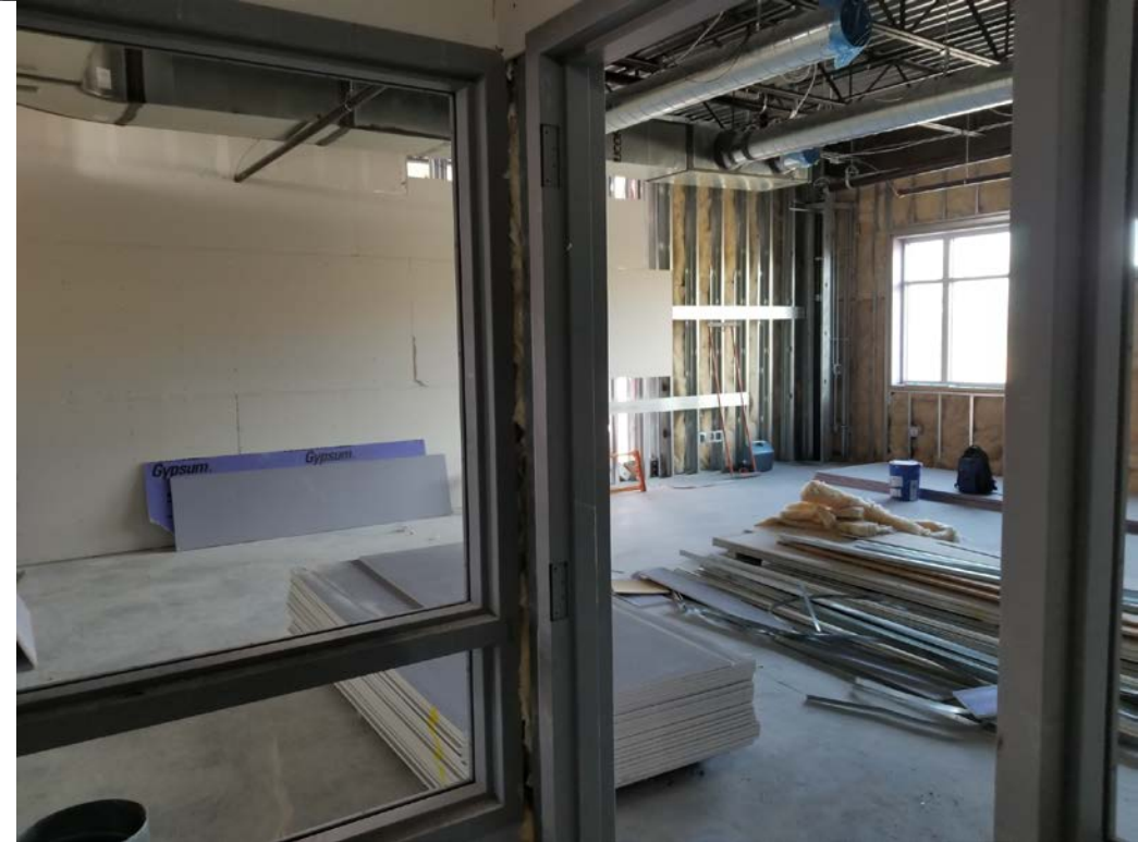
South Classroom Wing (upper level) – Classroom; Drywall being installed
