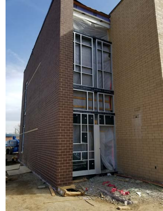
West Elevation; Frames installed on classroom wing staircases
