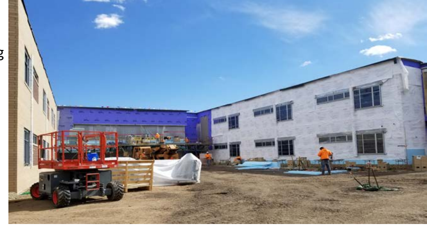
North Classroom Wing – Northwest Elevation; Brick, windows, and frames being installed.
