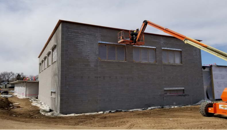
Front Entrance / Gym – Southeast Elevation; Brick, windows, and frames being installed; roof and parapet installation continues
