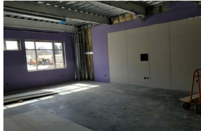
North Classroom Wing (lower level) - Classroom; Drywall being installed
