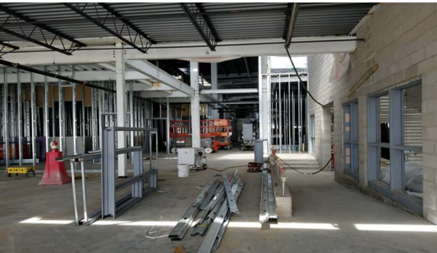
Grand Hall Main Entrance – North Facing View; Framing and HVAC being installed
