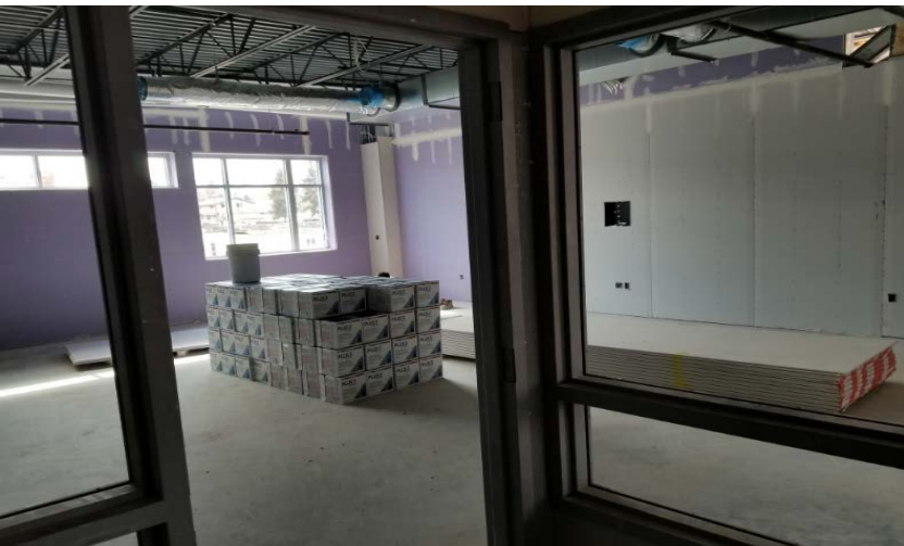
North Classroom Wing (upper level) – Classroom; Drywall and HVAC installed
