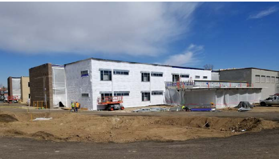
Front Entrance – Southwest Elevation; Windows and frames installed; Brick install; Roof and parapet installation continues
