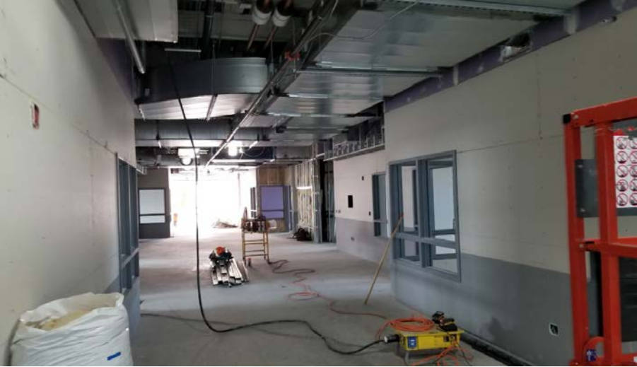
North Classroom Wing (upper level) – West Facing View; Drywall and HVAC installed; Framing for drywall soffit to begin
