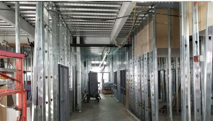
South Classroom Wing (lower level) –West Facing View; Framing, HVAC, and plumbing being installed
