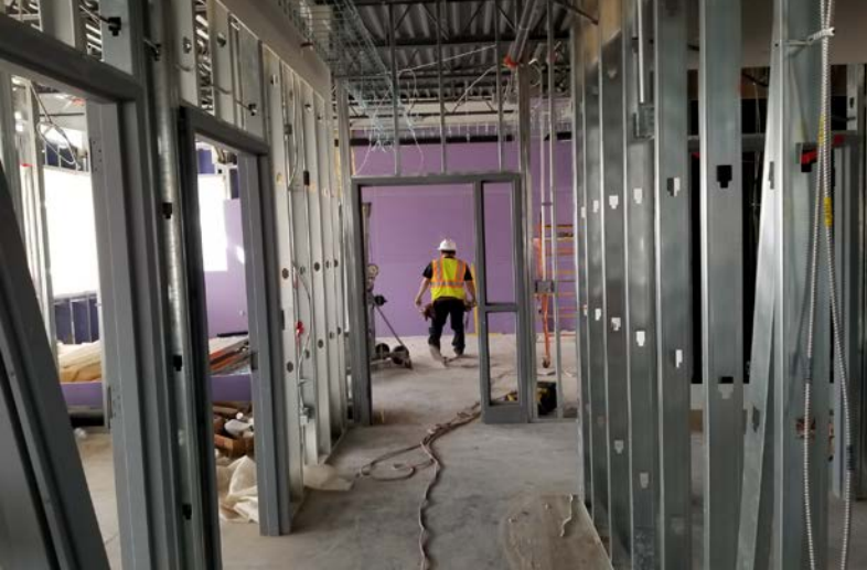
Office Area – West Facing View; Electrical, mechanical, insulation, and drywall being installed
