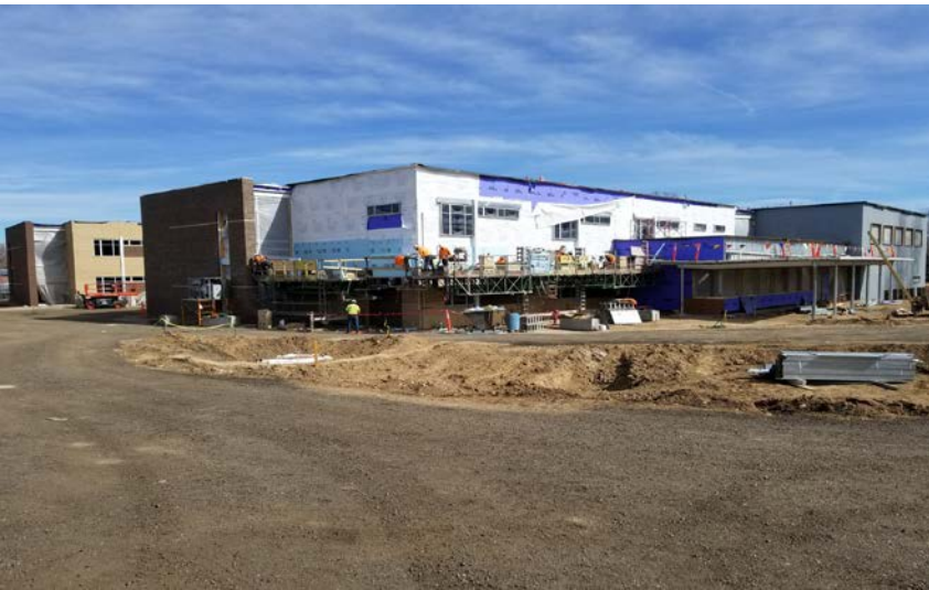
Front Entrance – Southwest Elevation; Brick, roof and parapet installation continues
